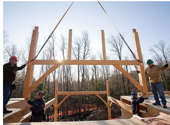
Figure 5.1 – Construction Crew Raising a Timber Frame (Source: Truini, J. (2007, March 22) Popular Mechanics: A House With No Nails: Building a Timber-Frame Home )
