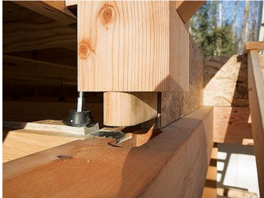
Figure 5.2 - CNC Cut Timber Joinery (Source: Truini, J. (2007, March 22) Popular Mechanics: A House With No Nails: Building a Timber-Frame Home )
