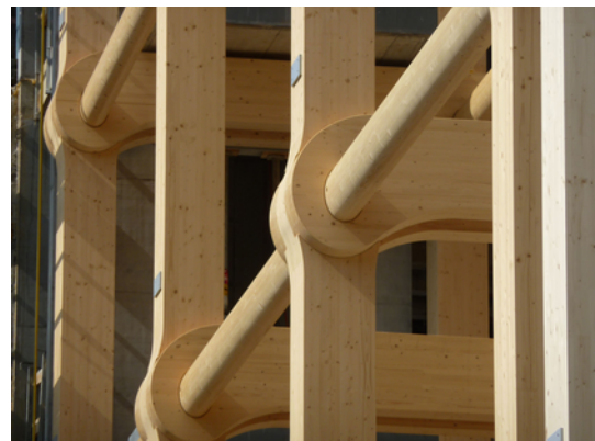
Figure 5.5 - Engineered wooden joint at the Tamedia office building © Shigeru Ban Architects
