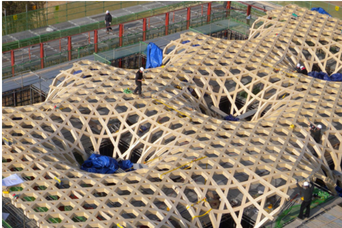
Figure 5.8 - Nine Bridges Clubhouse Roof Structure Under Construction © Shigeru Ban Architects
