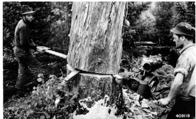
Figure 2.3 - Gasoline driven power saw. Tumble Creek fire near Detroit, Oregon. U.S. Forest Service Historic Photograph #409118
