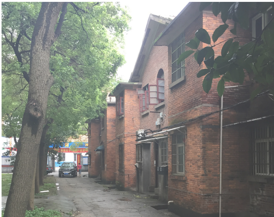
Fig 163, A old brick residential building that will soon be demolished in the city's Yueyang Pavilion area development plan. Photo in July, 2016.
