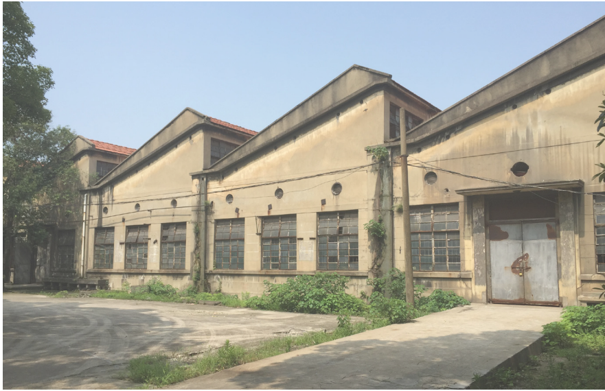
Fig 157, No.6 Workshop Building of 3517 Factory, Photo in 2016
