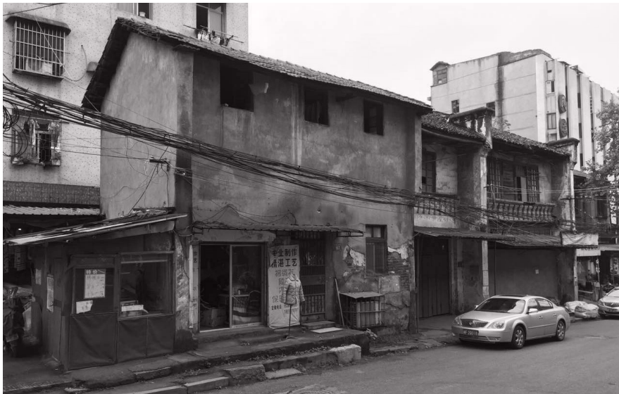
Fig 100, An residential house changed its first floor to a Tailor's shop, an informal expansion attached to its left side.
