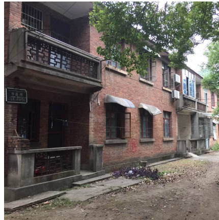
Fig 106, Self built entry space.
