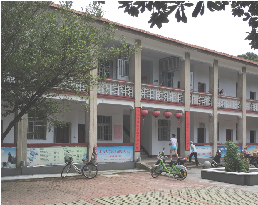
Fig 162, A typical old office building with each unit door opens to a public corridor on every floor.
