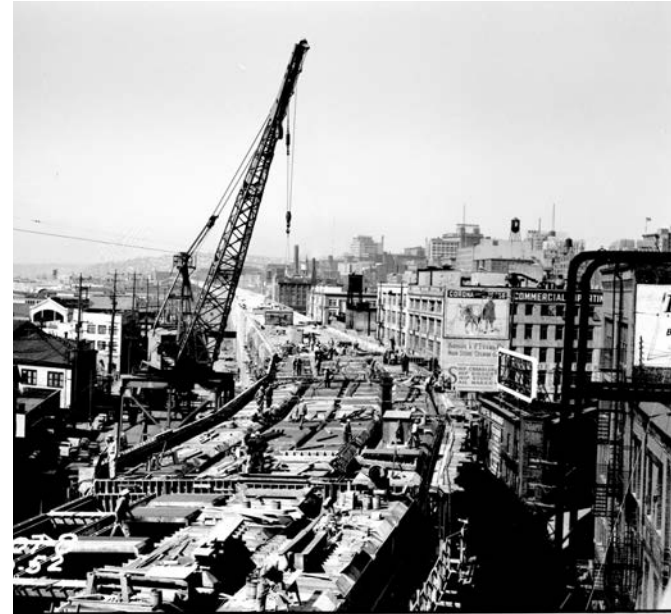
Figure 43 - Viaduct under construction Source: WSDOT
