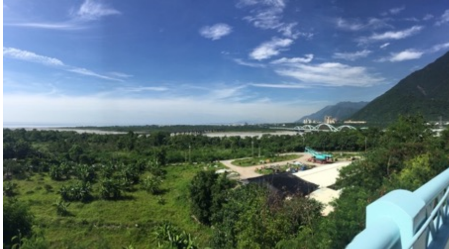
Overview of the Chongde site. Photo direction: north to south
