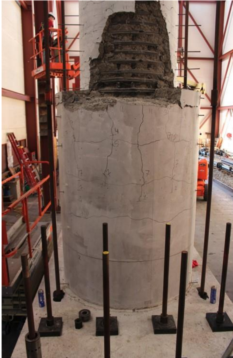
Figure 2.6: Photo of post-test damage in specimen UCSD-2 (Murcia-Delso et al. 2013)
