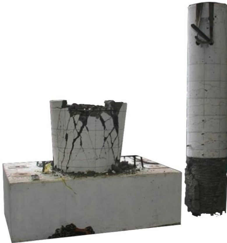
Figure 2.10: Photo of post-test damage in specimen DS-2 (Tran 2015)
