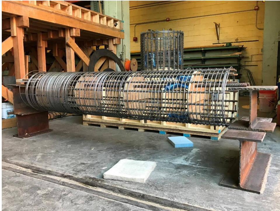
Figure B.2: Column reinforcement cage in progress
