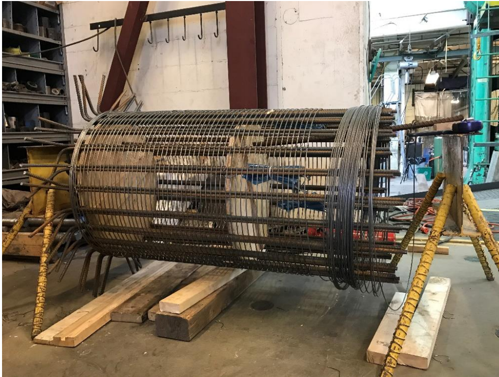
Figure B.1: Shaft reinforcement cage in progress
