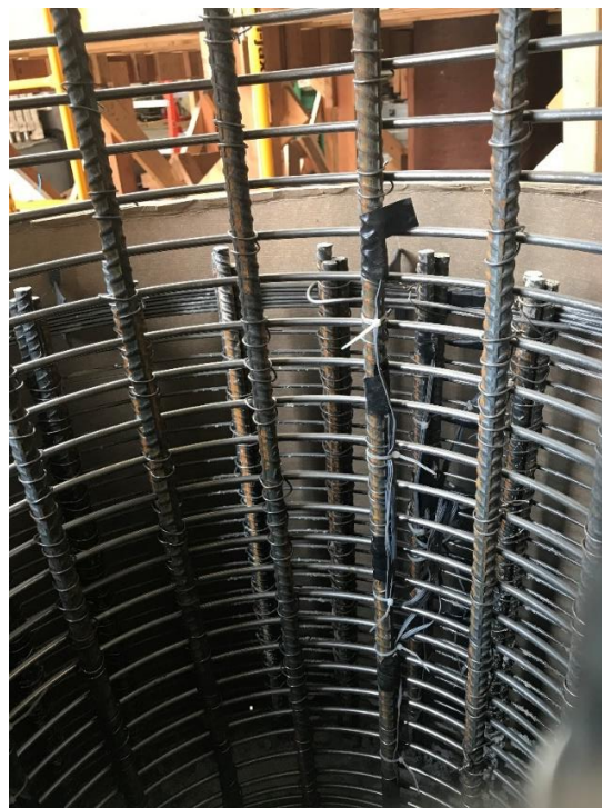
Figure B.5: Covered strain gauges on column longitudinal bar (north bar)
