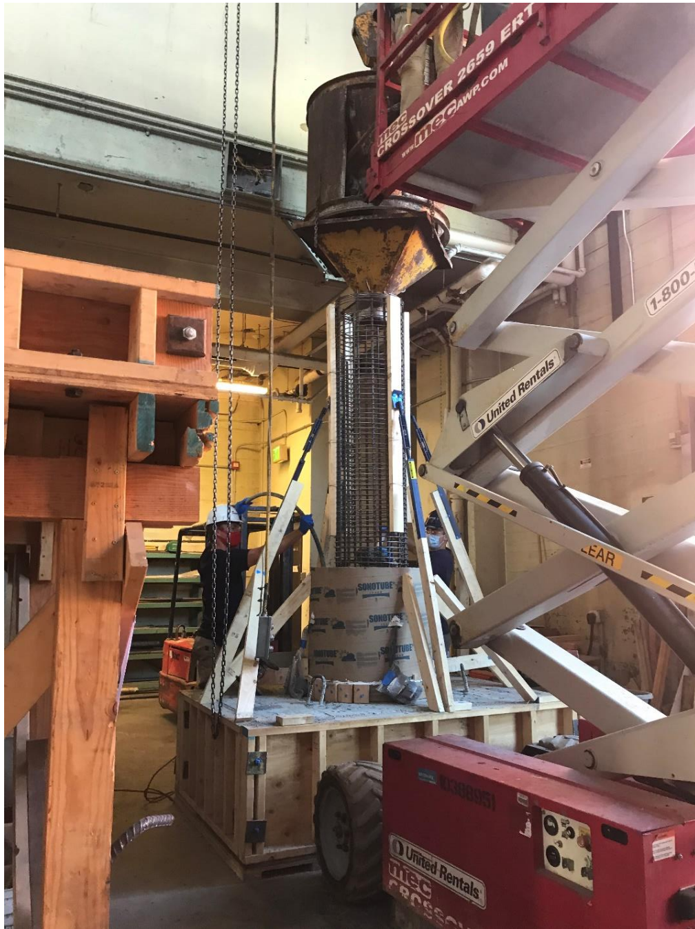
Figure B.6: Concrete placement for the shaft (pour #2)
