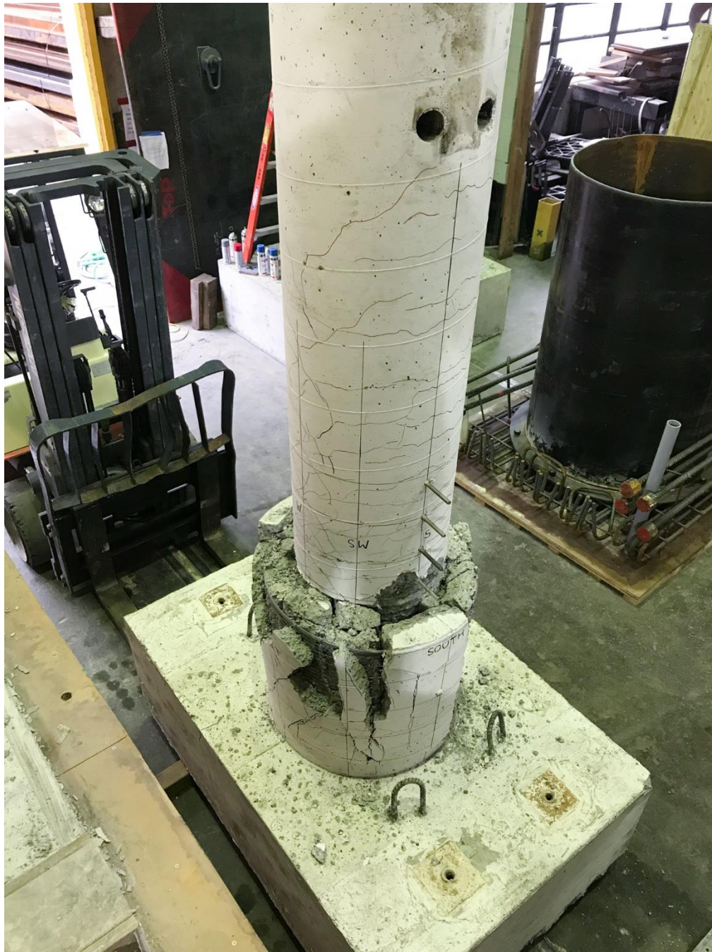
Figure D.5: Overhead angled view of specimen from southwest (post-test)
