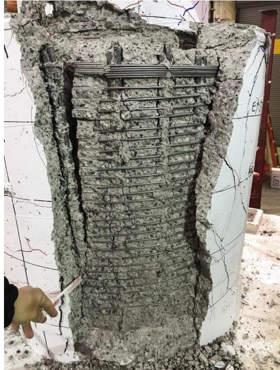
(d) Transverse reinforcement fractured down to the level of the pencil (height of shaft = 30 in.)
