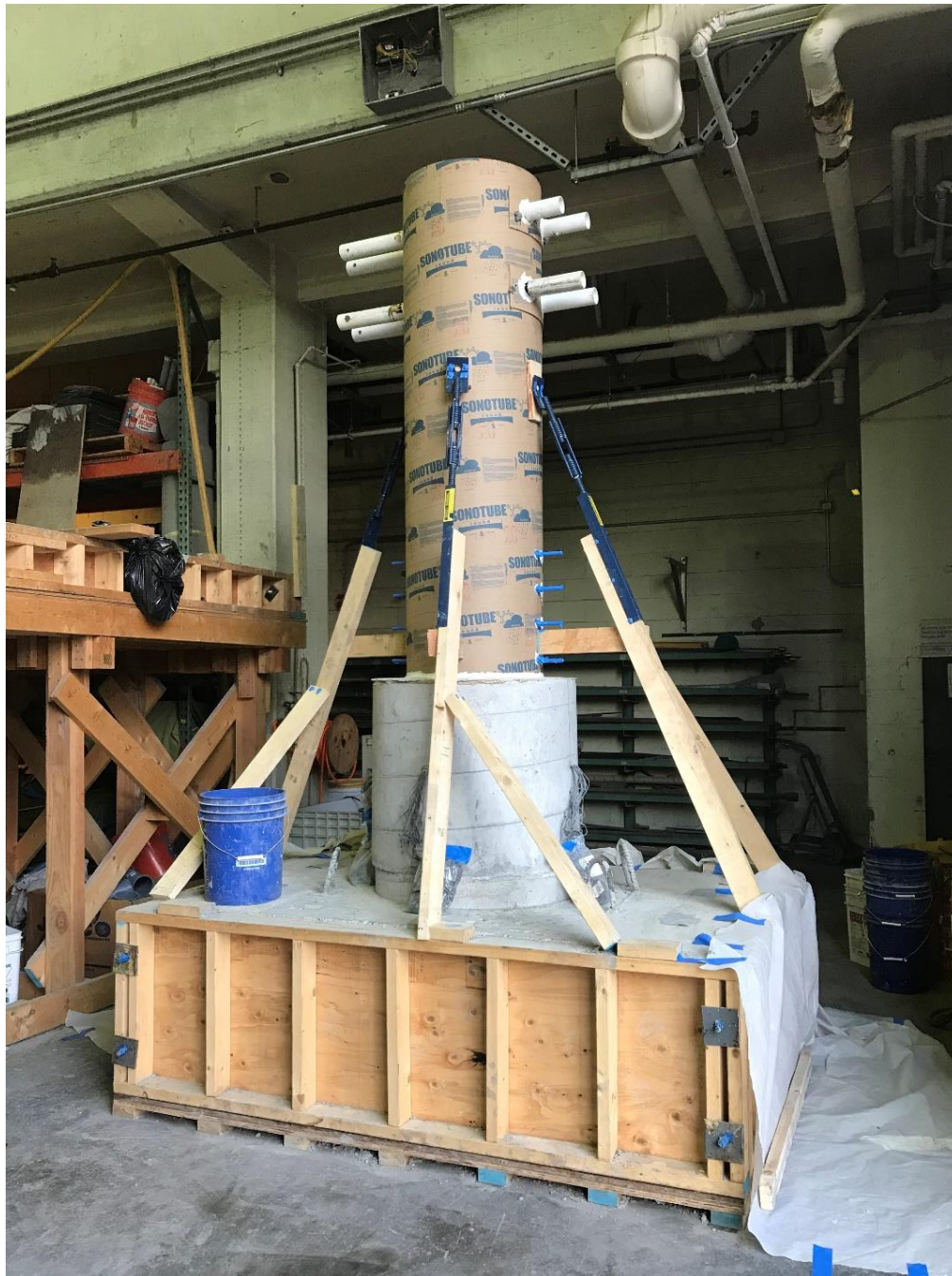
Figure B.7: Formwork and embedded items for the column
