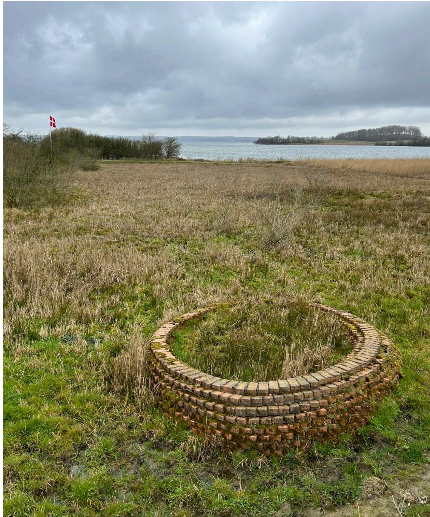
Figure 6.16 Stormwater structure built from salvaged bricks near Catherinesminde Teglvaerk in Broager, Denmark (Photo by author)
