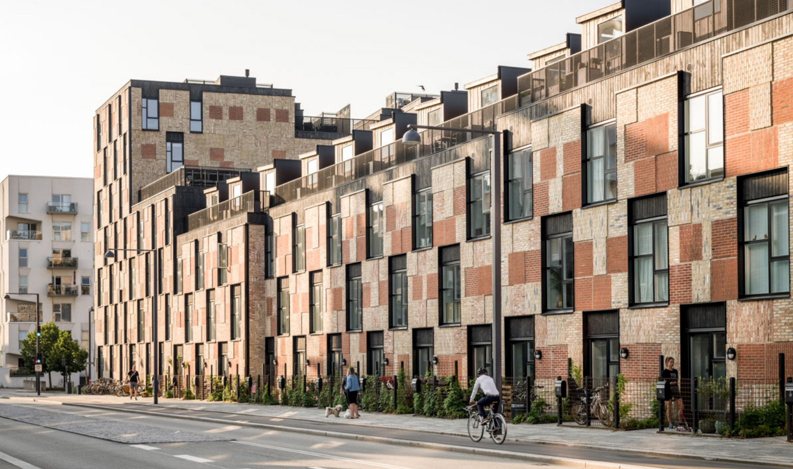
Figure 7.1 Exterior photograph of the Resource Rows repurposed masonry facade. Completed in 2020 by Lendager Architects in Copenhagen (Photo courtesy of Lendager Architects)
