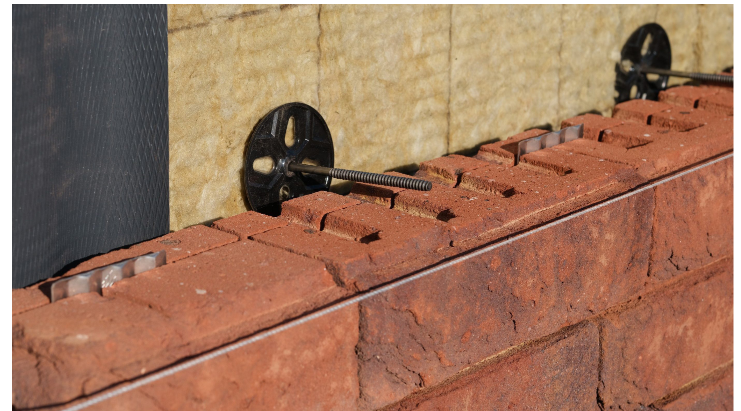
Figure 7.10 ClickBrick installation detail with masonry anchors tied back through a layer of continuous exterior insulation (Photo courtesy of Wienerberger)
