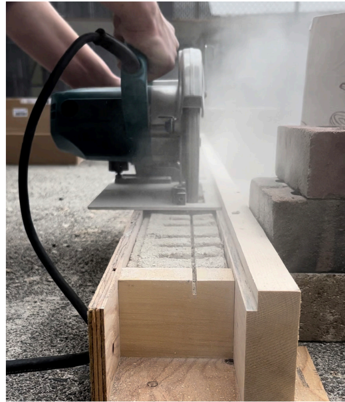
Final Channel Cuts
