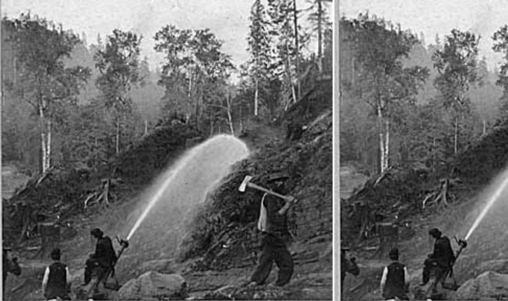
Figure 3.1 Clay mining with high pressure hoses in 1890's Renton, WA (Photo courtesy of Renton History Museum and Museum of History & Industry)
