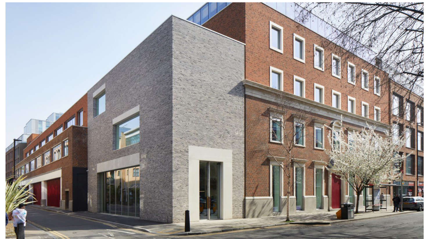
Figure 7.5 Waste Based Bricks utilized as an exterior facade in the new Technique office space in Clerkenwell, London by Buckley Gray Yeoman Architects. The bricks are responsible for upcycling 22,080 kg of waste material (Photo courtesy of Jack Hobhouse)
