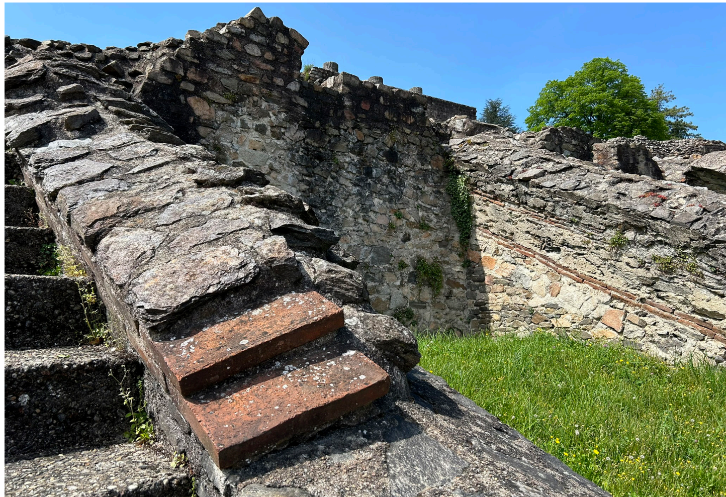
Figure 2.3 Remains of a brick and stone wall system at the Roman theatre complex of Fourvière in Lyon, France, dating back to the 1st century B.C.E. Square shaped bricks were used here as setting courses between wider masses of stone set in concrete, taking advantage of the fired material's more precise dimensions in complicated construction areas like the archway shown here (Photo by author)
