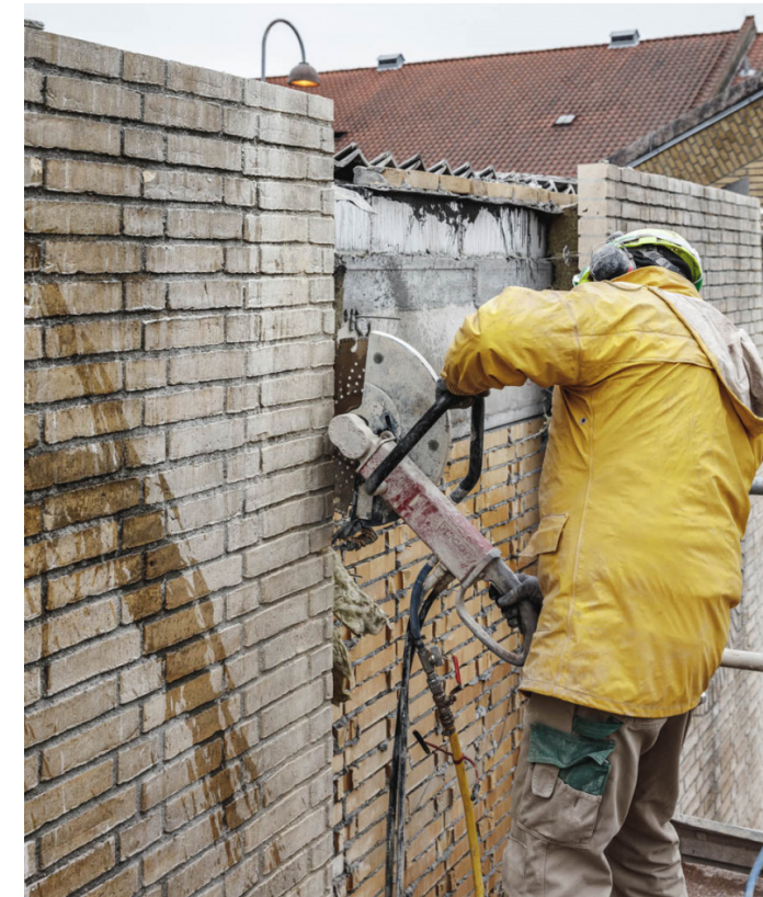
Figure 7.2 Existing masonry walls at the former Carlsberg factory permanently bound with cement mortar are cut into panels and repurposed into a quilted facade at Resource Rows in Copenhagen, Denmark by Lendager Architects (Photo courtesy of Lendager Architects)
