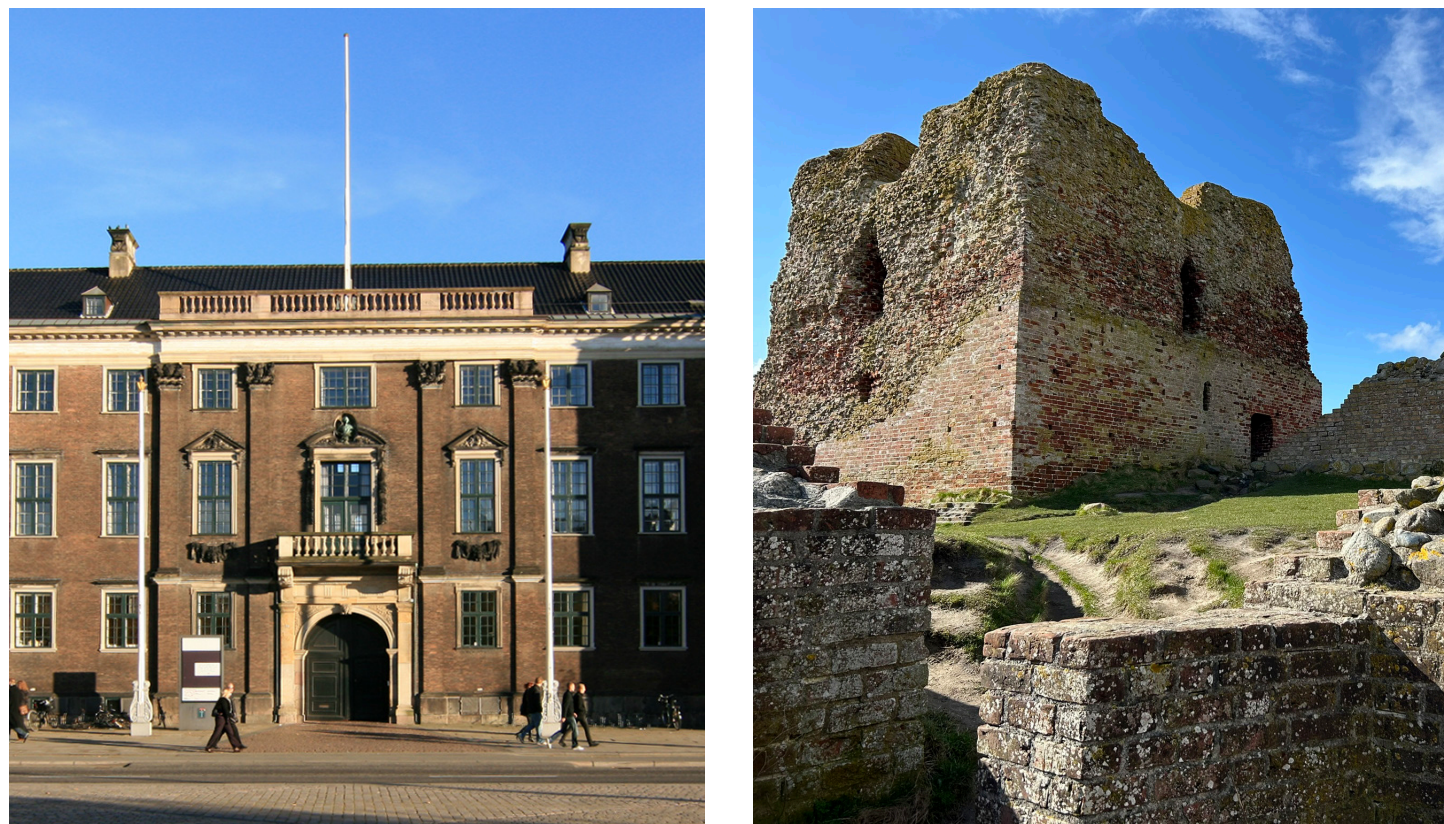
Figure 1.7 (left) Charlottenborg Palace from Kongens Nytorv square in Copenhagen, Denmark. The palace was constructed in the 18th century, but is composed of salvaged bricks from 14th century Kalø Castle in Figure 1.8 (right) (Photos by author)
