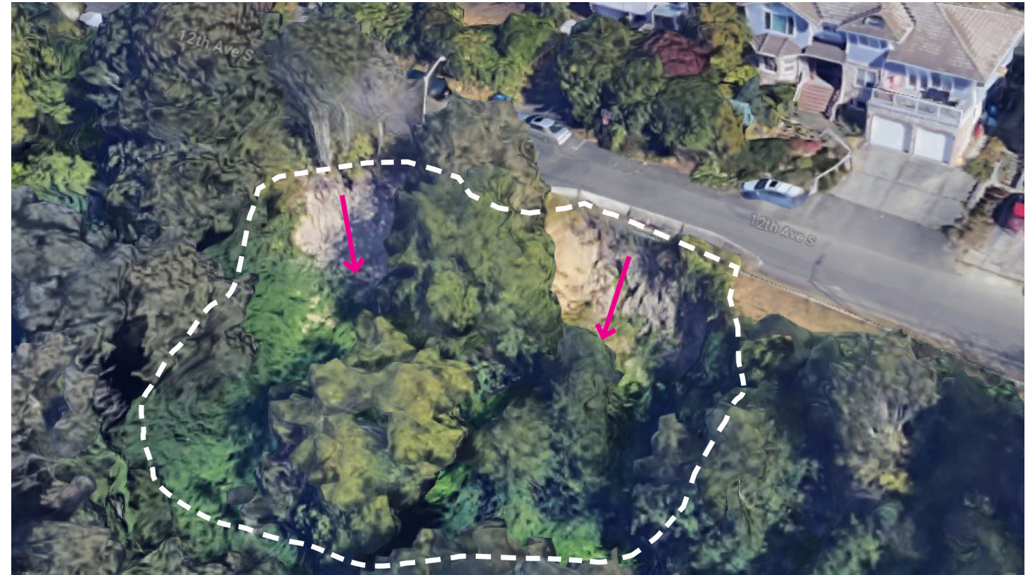
Figure 3.11 Aerial photograph of present day conditions at the former site of the Beacon Hill Clay Mine. Steep surface erosion is visibly approaching the adjacent residential neighborhood (Aerial photo adapted from Google Maps)
