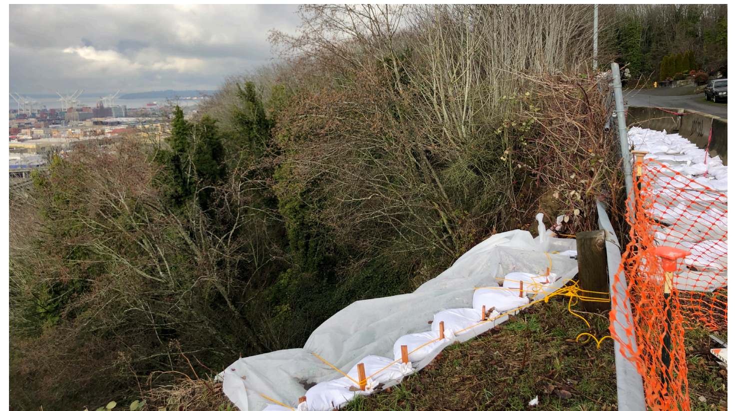
Figure 3.12 Evidence of hillside erosion at the present day location of the Builders Brick clay pit is posing an increasing threat to adjacent residents (Photo by author)
