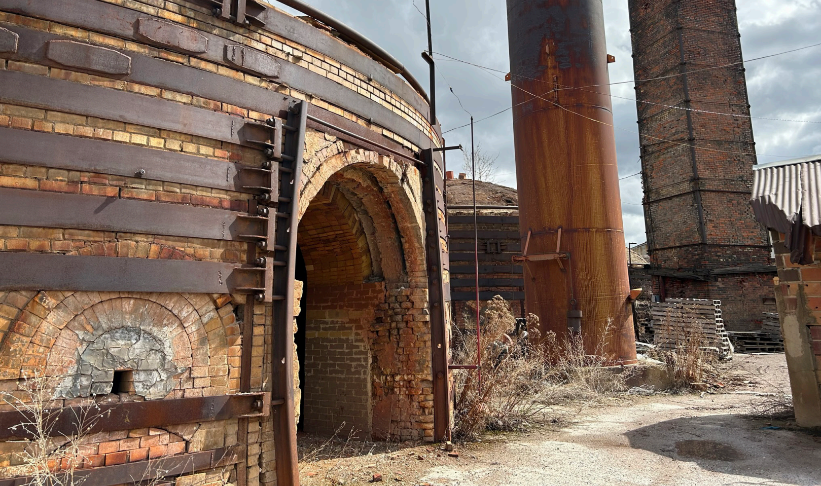
Figure 4.1 Retired beehive kilns at the present-day Mutual Materials brick production facility in Mica, WA (Photo by author)
