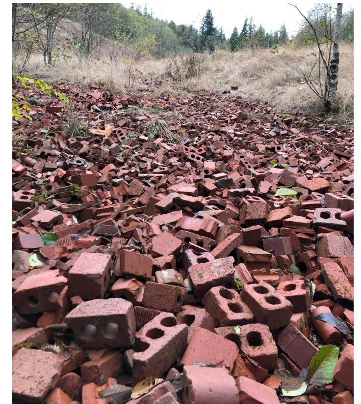
Figure 6.5 Brick clinker pile serves as a filter to surface water runoff heading downslope towards the settling pond (Photo by author)
