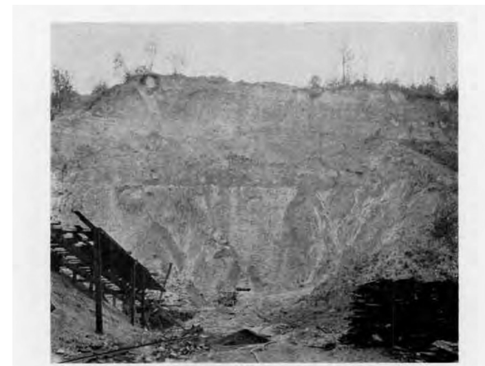
Figure 3.8 The Beacon Hill clay mine, operated by Builder’s Brick Company until the construction of I-5 in the late 1950’s (Photo courtesy of Solon Shedd)
