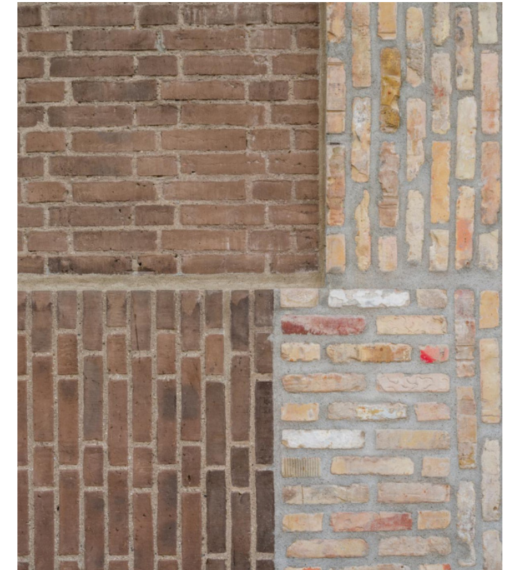
Figure 7.2 Existing masonry walls at the former Carlsberg factory permanently bound with cement mortar are cut into panels and repurposed into a quilted facade at Resource Rows in Copenhagen, Denmark by Lendager Architects (Photo courtesy of Lendager Architects)
