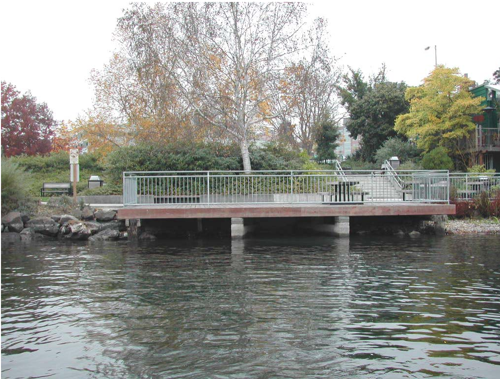
Figure 6. Overwater platform shading the shoreline.
