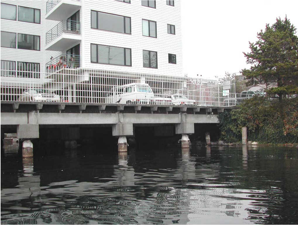
Figure 5. Overwater structure shading the shoreline.
