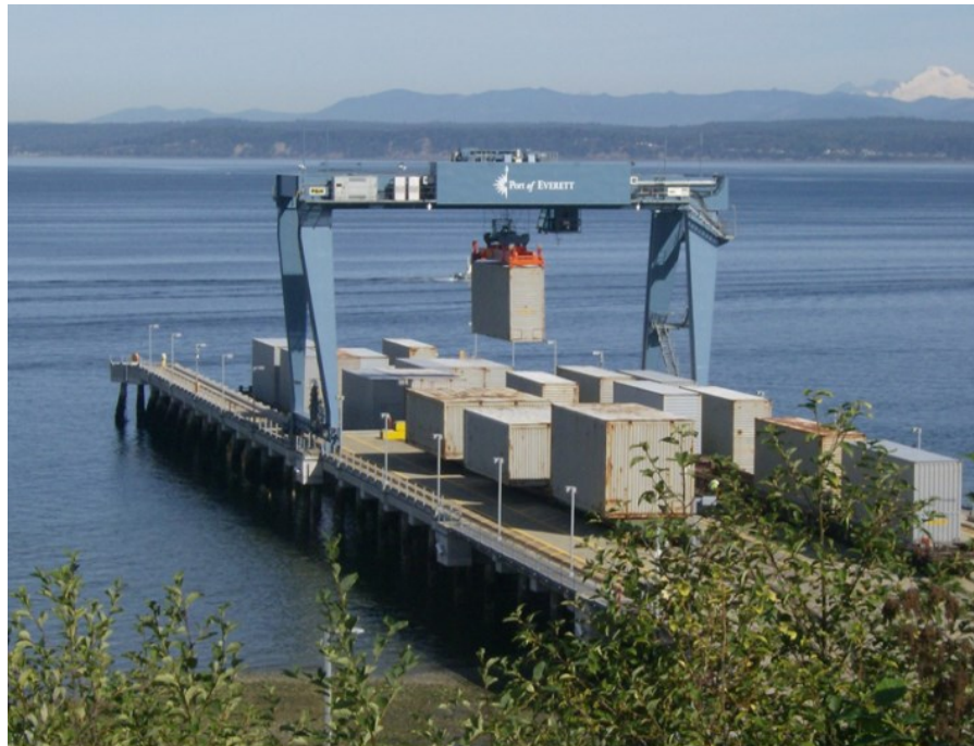
Figure 3 – Barge terminal at Mukilteo.
