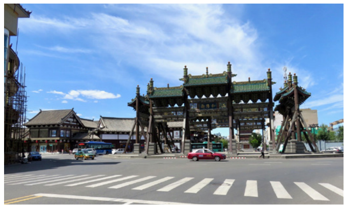
Figure 5.43d: Four Archways, Datong (Ho, 2019).
