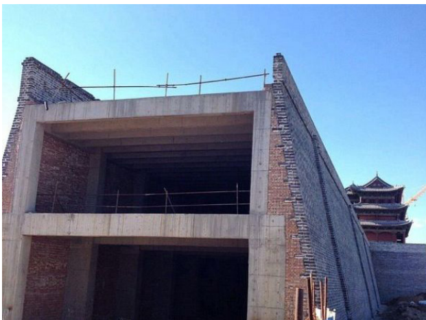
Figure 5.32e: (left) Concrete framework for reconstructing City wall. (Source: https://pic2.zhimg.com/41d7214ad6193d3cf6d4965c4f1aacbd_b.jpg ); (right) Reconstruction of city wall, Datong, 2010. (Source: Sun, G. (2011). Love in Datong .)
