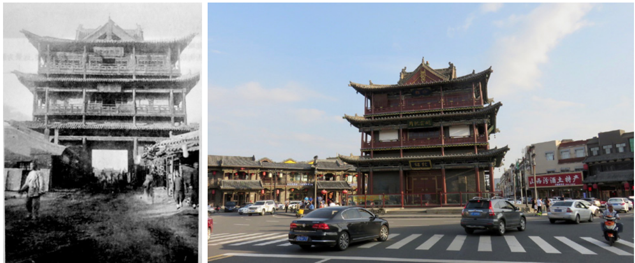
Figure 5.33b: (left) Drum Tower, 1907 (E. Chavannes) (Source: Zhang, C. (2009). Datong Ancient City and vernacular dwellings . Fig.4); (right) Drum Tower after restoration (Ho, 2019).
