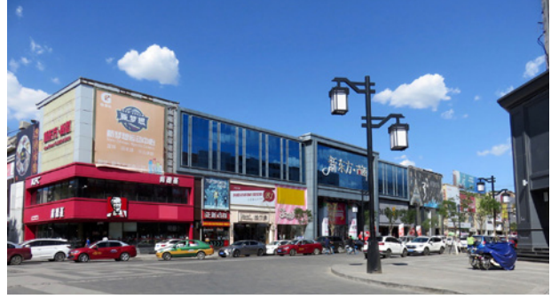
Figure 5.36b: Modern commercial buildings, Jiaochang St., Datong (Ho, 2019).
