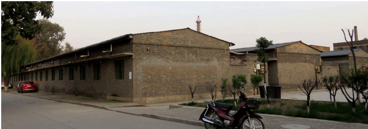
Figure 5.29a: Factory, Diesel Engine Plant, Pingyao ( Ho , 2019).
