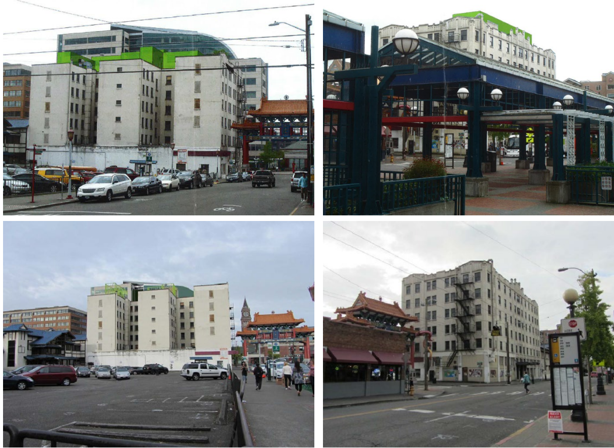
Figure 6– Penthouse Renovation at the Publix Hotel
