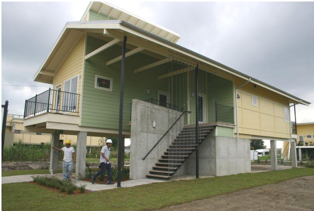
Figure22. A hurricane-resistant home going up in the Lower 9th Ward community in New Orleans .Brad Pitt's Make It Right Foundation. (2014/March) .Retrieved from URL: http://kathyprice.typepad.com/dispatch_from_new_orleans/lower_ninth_ward/ .Accessed: 2014-06-09. (Archived by WebCite® at http://www.webcitation.org/6PtXqC2wX )
