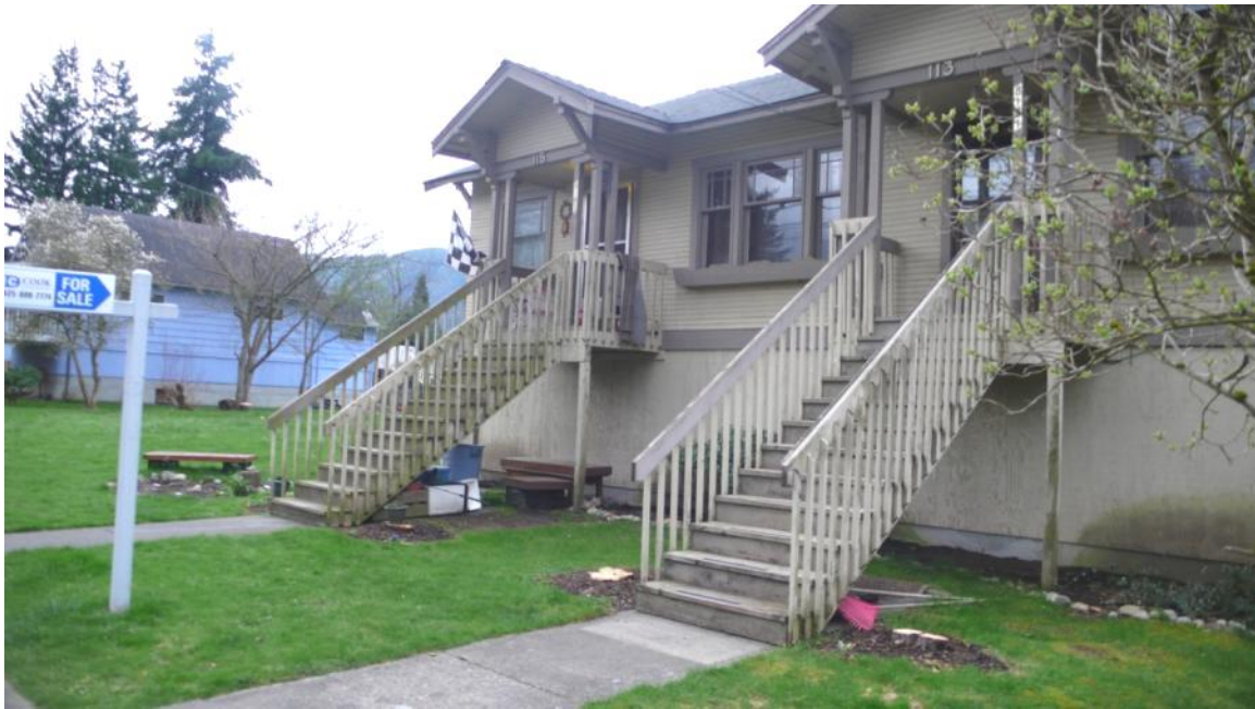
Figure50.Elevated houses along Snoqualmie River. Shot by Pin-hao,Huang.(March.2014).
