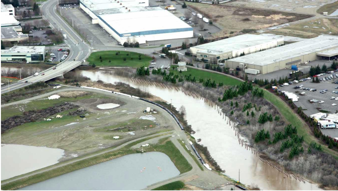
Figure16. Boeing Levee, Adapted from “GREEN RIVER PROJECTS” by City of Kent, 27 April 2012, p006
