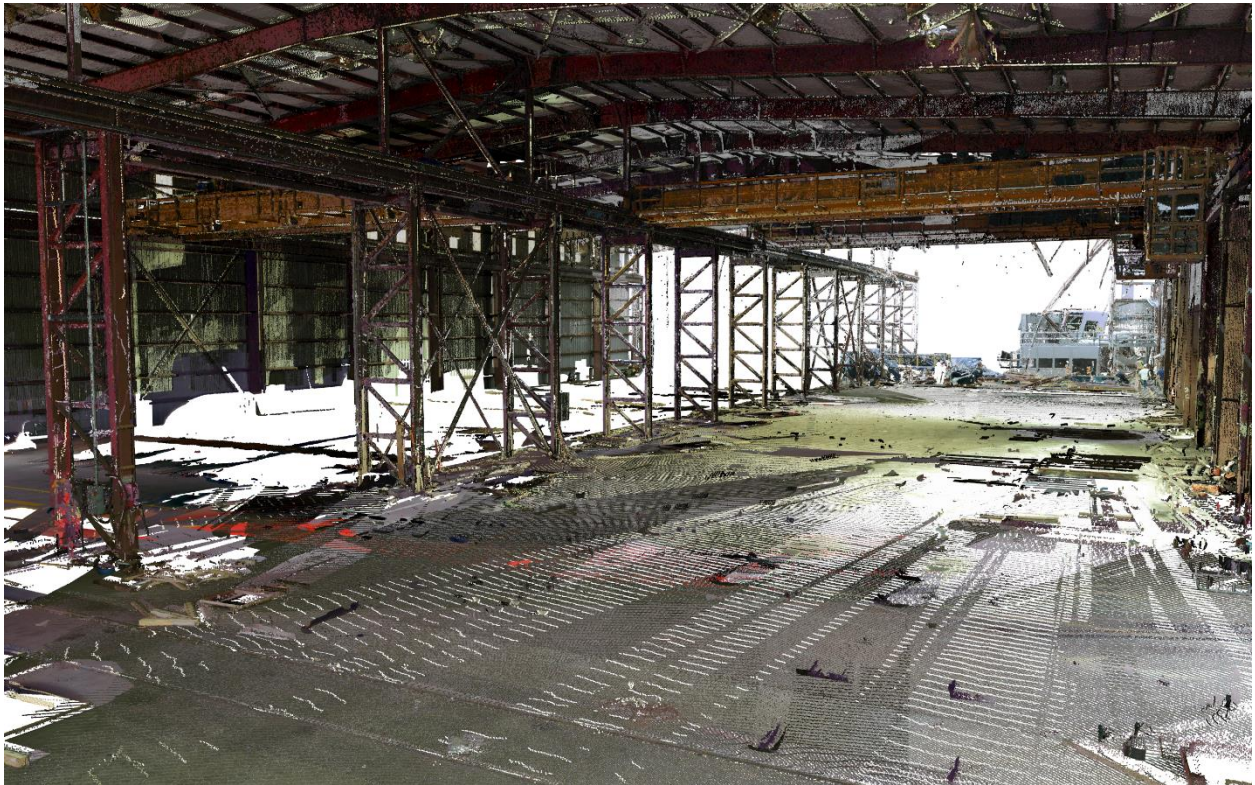
Figure 4.44. Inside view after cleaning with both XR3 and BLK360
