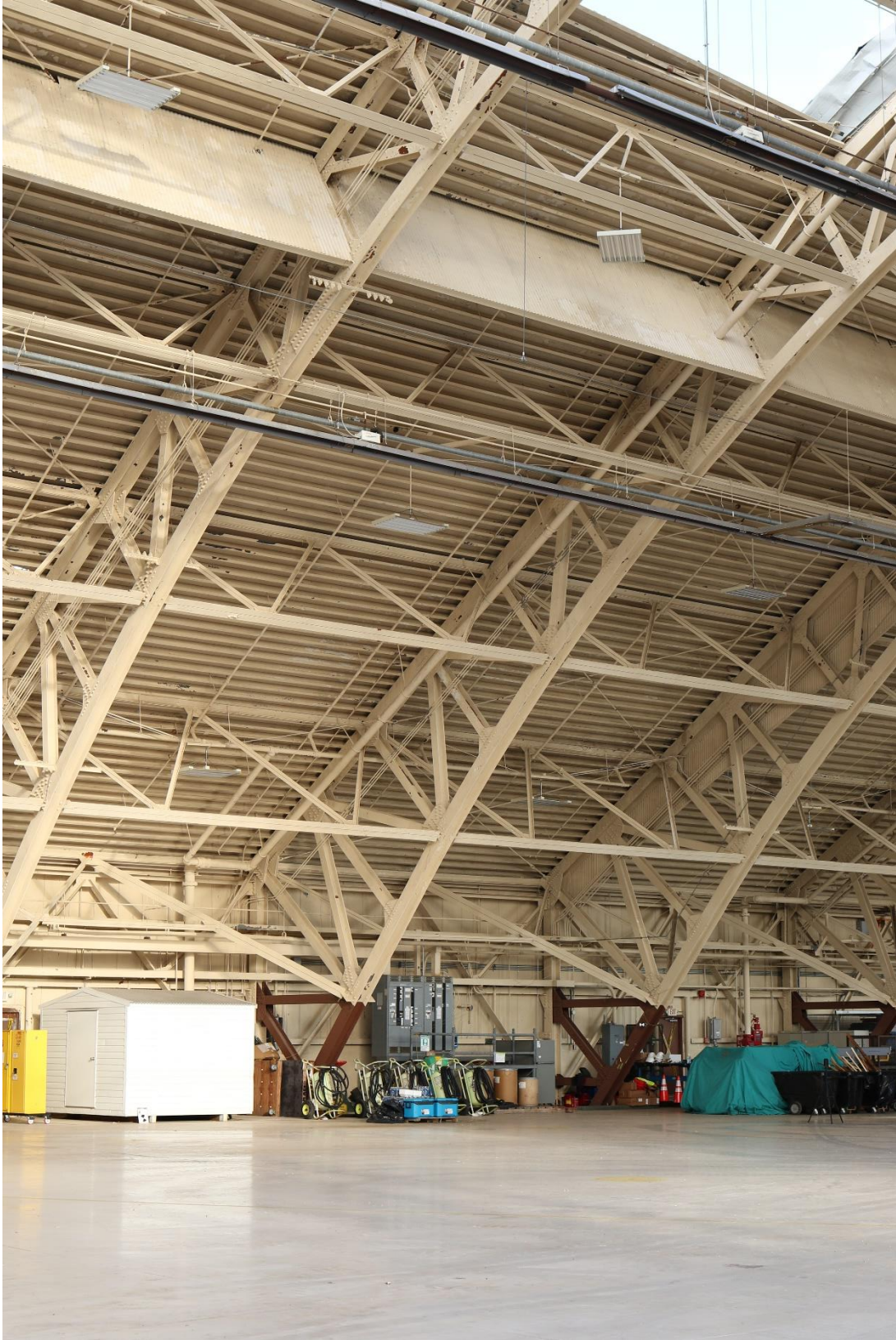
Figure 3.21. Roof framing in Hangar 5.
