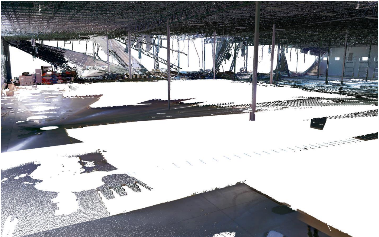
Figure 4.32. Inside view after cleaning with both XR3 and BLK360
