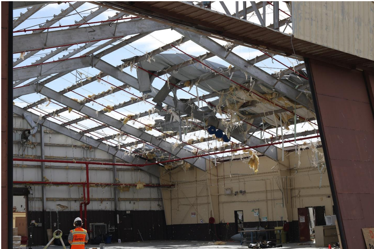
Figure 3.24. The roof system of Building 316.
