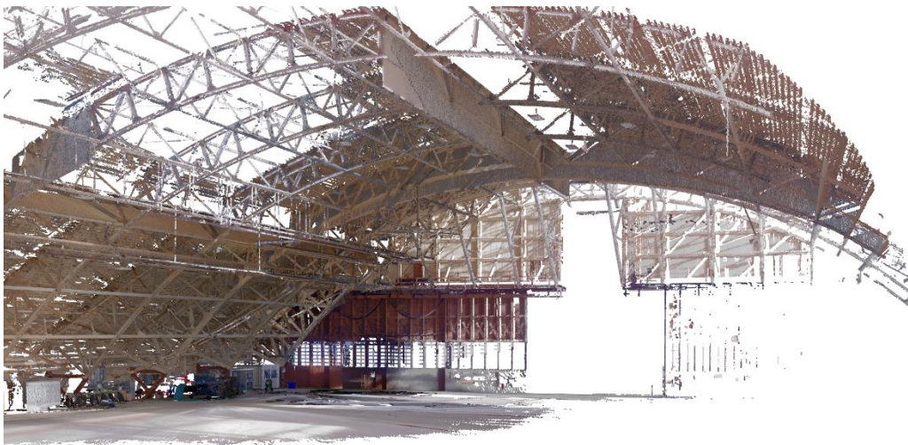
Figure 4.51. Inside view before cleaning showing only BLK360 data.
