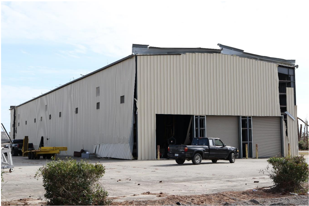
Figure 3.26. Front view of Building 333.
