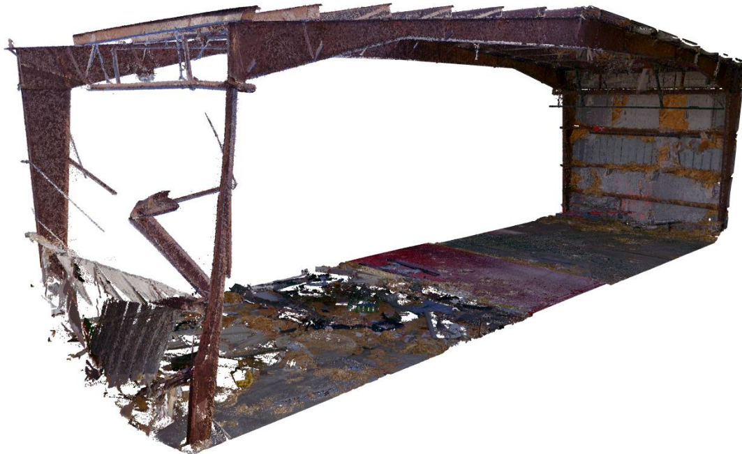
Figure 4.84. A single bay from Building 375.
