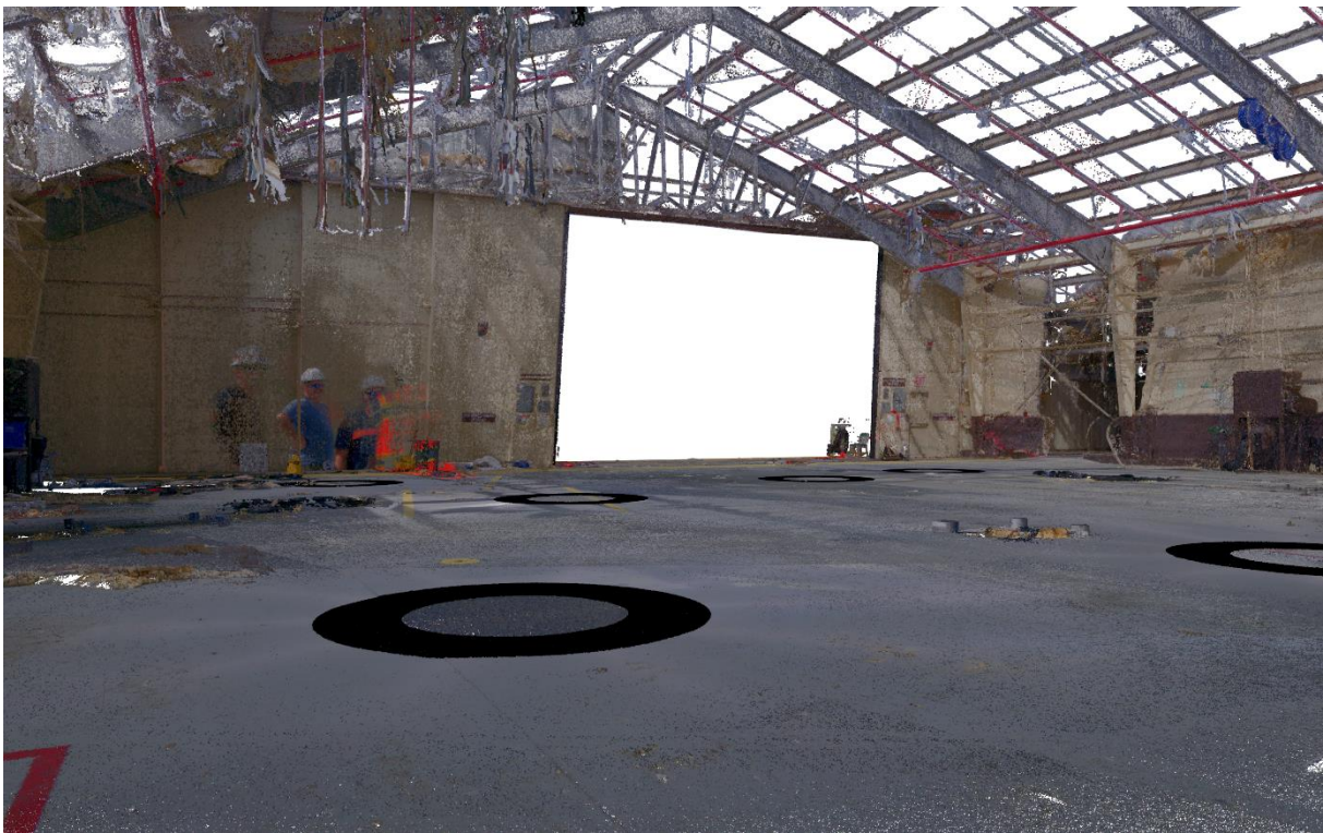
Figure 4.64. Inside view after cleaning showing only BLK360 data.
