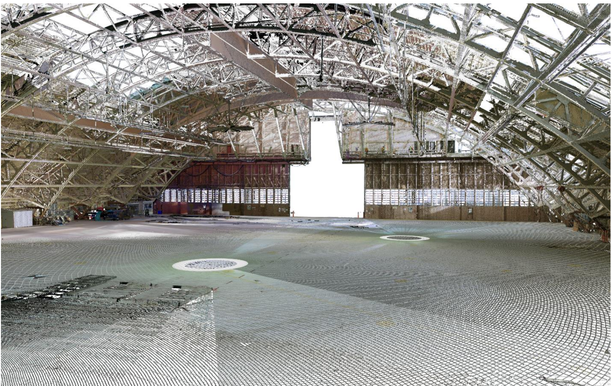
Figure 4.56. Inside view after cleaning with both XR3 and BLK360
