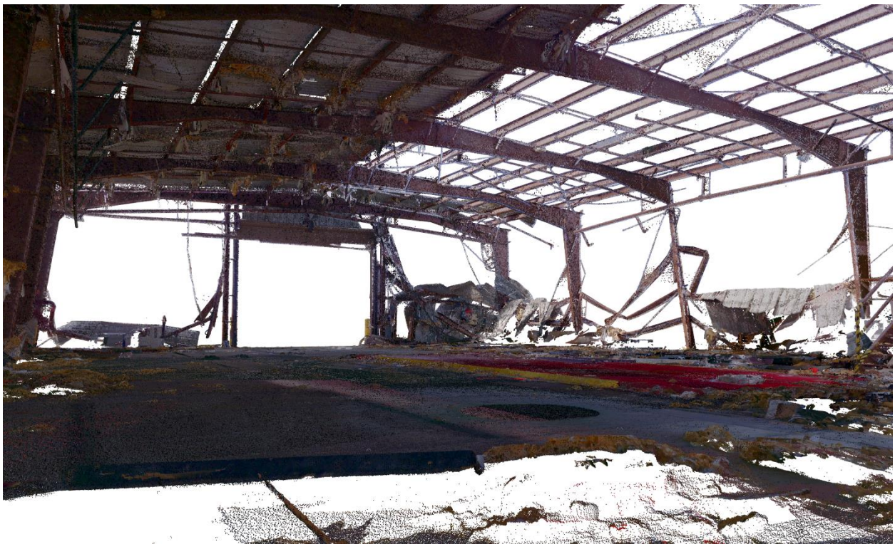
Figure 4.80. Inside view after cleaning showing only BLK360 data.
