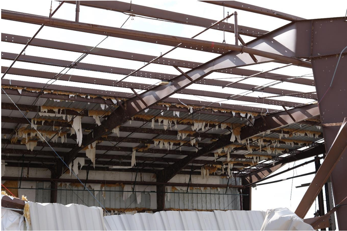
Figure 3.29. The framing system in Building 375.
