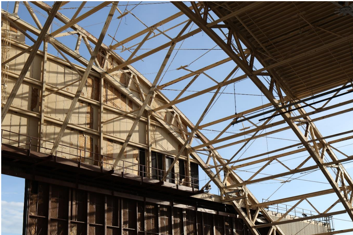
Figure 3.20. Roof framing in Hangar 5.
