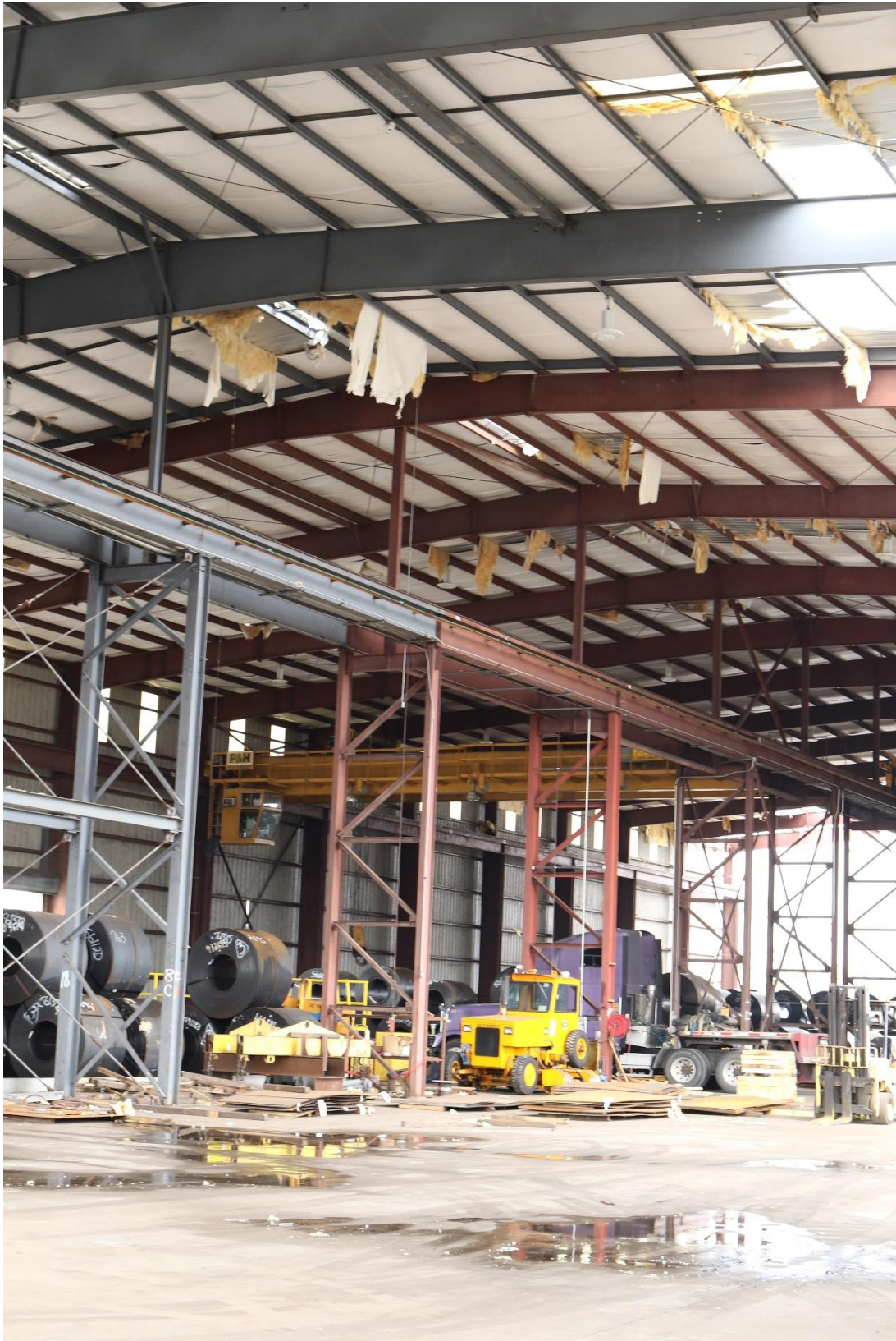
Figure 3.17. The framing system of Cargill Distribution Center.
