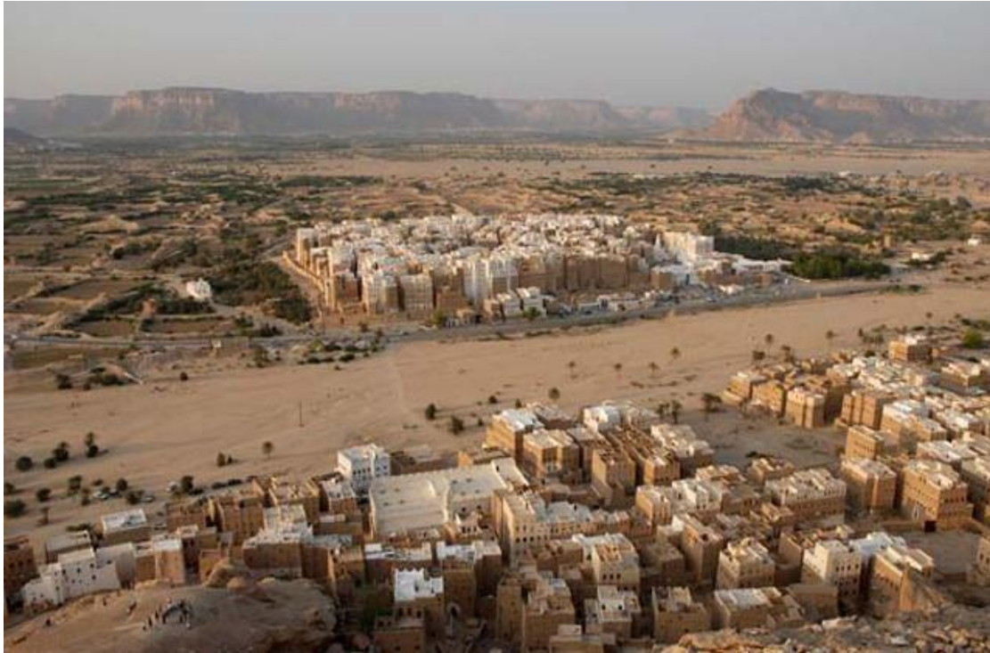
FIG 2.32. Aerial view of Shibam, where the AKAAs reads conservation not as the preservation of an image but as the maintenance of a living urban platform. The city's value lies in the systems that allow its dense mud-brick fabric to remain inhabited.
