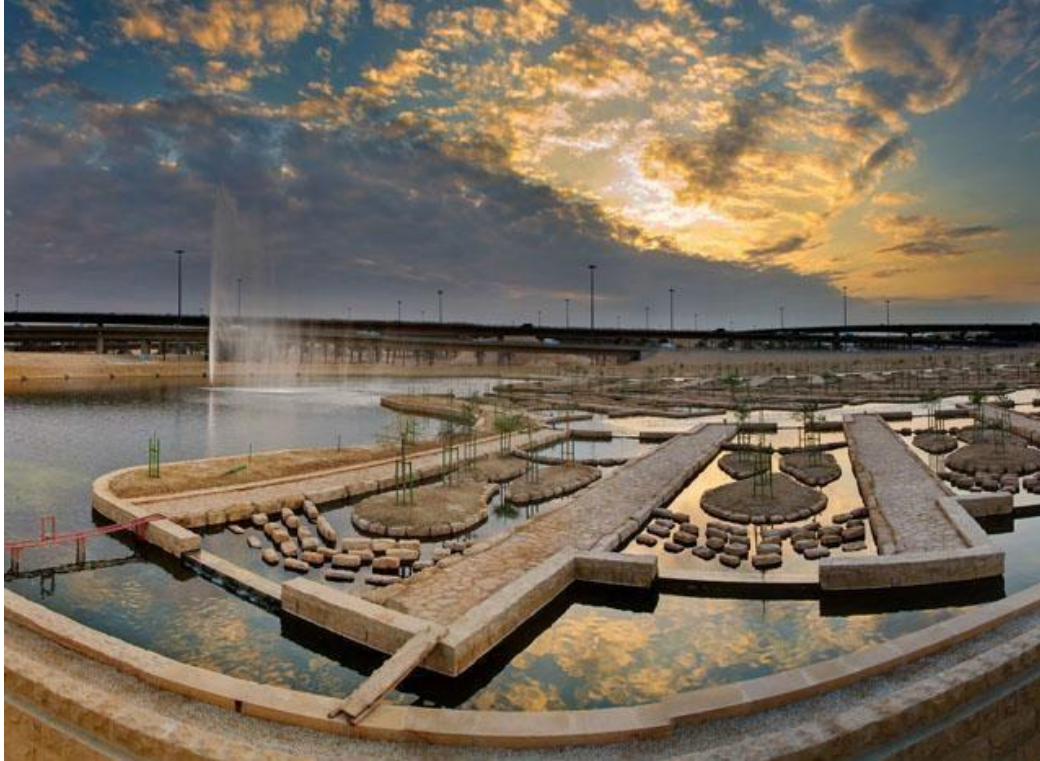
FIG 2.4. Bio-remediation facilities in Wadi Hanifa, where water treatment, flood mediation, and public landscape design are integrated. The project makes technical infrastructure visible as part of an ethic of stewardship and repair.
