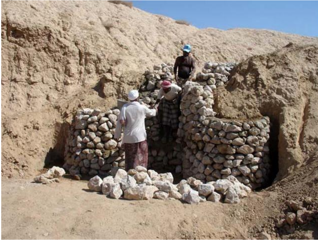
FIG 2.34. Construction of the Spate Irrigation System in Shibam. The image shows that conservation extends beyond walls and towers to the water infrastructures that sustain the city's economy, agriculture, and settlement life.
