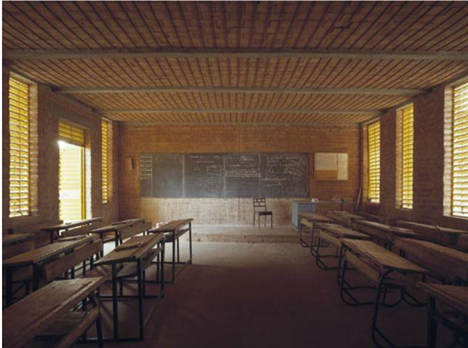
FIG 2.15. Interior of Gando Primary School, showing long shutters that provide natural light and ventilation. The classroom's comfort is produced through low-cost environmental design rather than mechanical systems, linking pedagogy to climatic adaptation.
