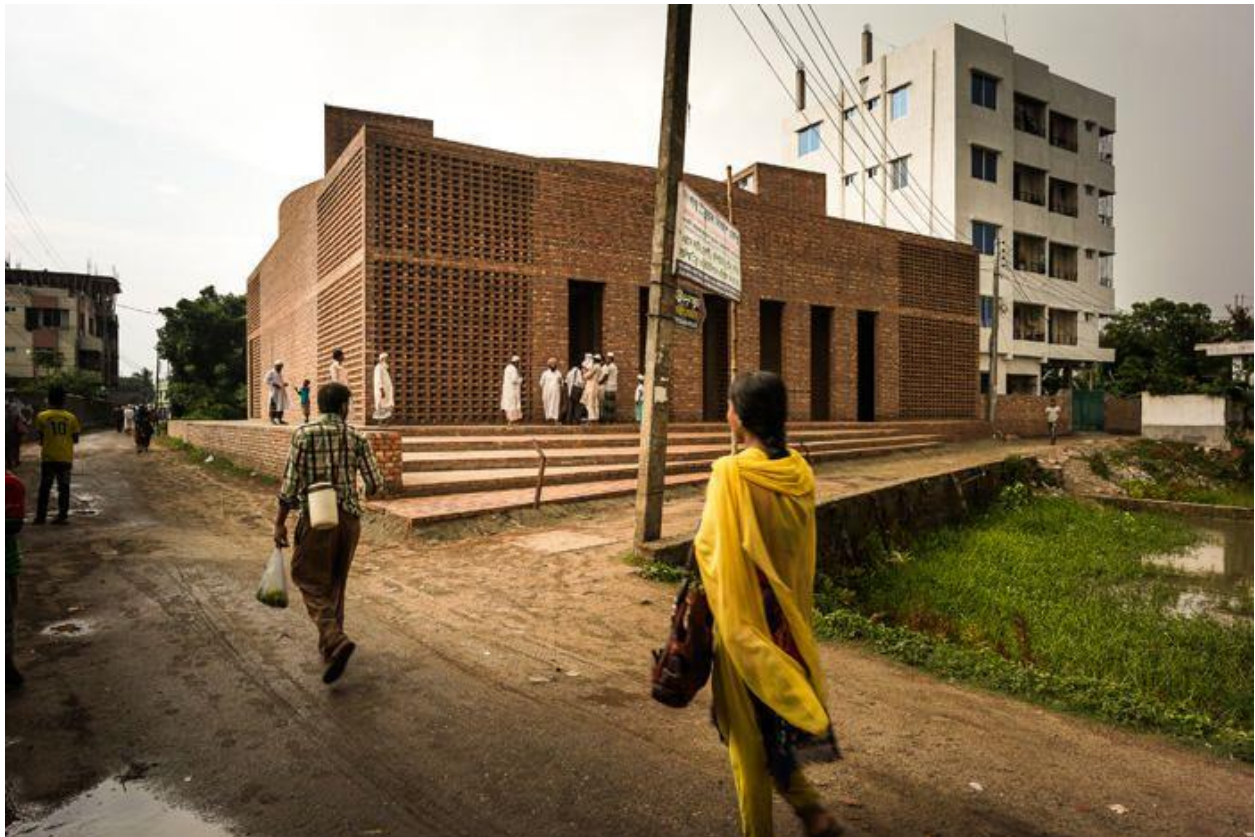
FIG 2.18. Exterior view of Bait ur Rouf Mosque, whose restrained brick volume rejects iconic mosque signifiers while preserving the mosque as a porous neighborhood institution. The project shifts Islamic architectural expression from dome and minaret to light, material, threshold, and shared use.
