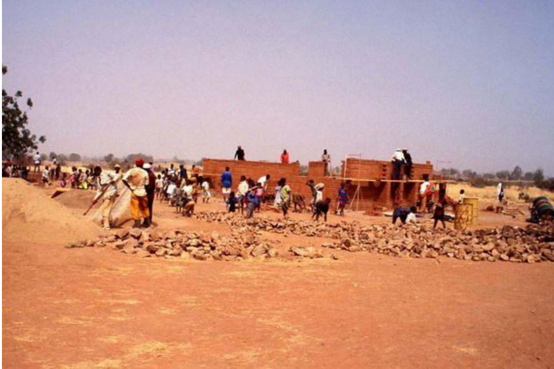
FIG 2.17. Construction view of Gando Primary School, emphasizing the community labor and technical experimentation behind the project. The image complicates any romantic reading of vernacular simplicity by showing the school as a hybrid of local labor, modern education, and careful material technique.
