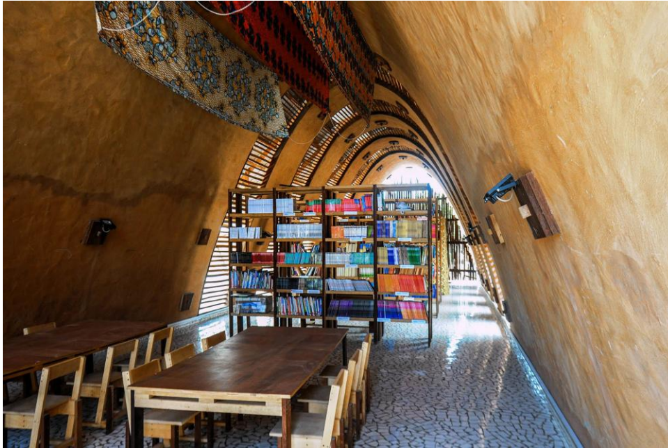
FIG 2.24. Clay construction, latticework, and vaulting at CEM Kamanar act together as a passive cooling system. The image shows how material form becomes environmental performance and architectural evidence.
