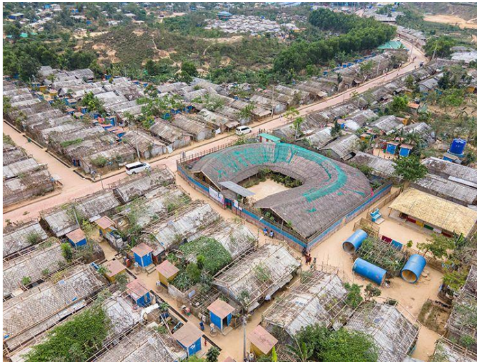
FIG 2.11. Aerial view of the community spaces in the Rohingya Refugee Response, Cox's Bazar. The project demonstrates how architecture can protect dignity and communal life under conditions of emergency and displacement.
