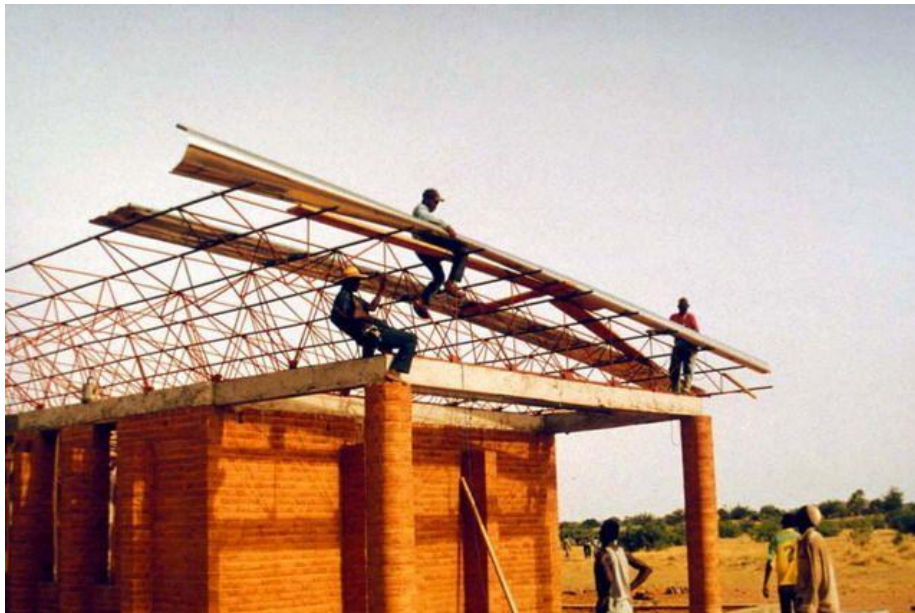
FIG 2.16 Workers assembling roof trusses during construction of Gando Primary School. The image foregrounds construction as civic training, showing how the project's process produced transferable skills alongside a school building.
