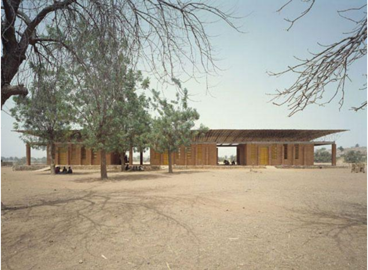
FIG. 2.14. Southern façade of Gando Primary School, where shaded thresholds, earthen walls, and simple assemblies make climate intelligence legible as civic capacity. The school’s architectural value lies not only in form but in its ability to be built, maintained, and extended by the community.
