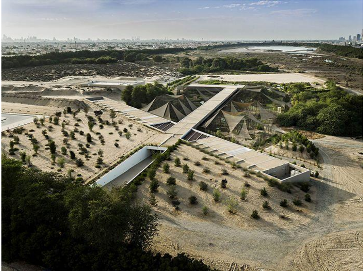
FIG 2.5. Aerial view of the Wasit Wetlands Centre, where the building's low profile allows the restored habitat to become the primary architectural presence. Its self-effacing form shifts attention from object-making to ecological recovery.
