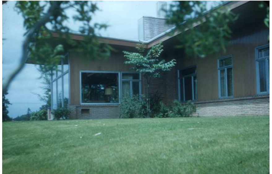
2.19 Raymond Huff house, designed 1948, exterior view. Photograph by Robert Reichert, c. 1960. (UW College of Built Environments Visual Resources Collection).
