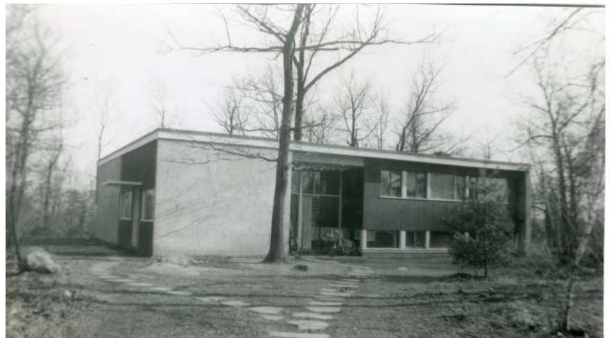
2.40 Photograph taken by Reichert of the Jean and Norman Fletcher house (the architect's own home), Six Moon Hill, 1951. (Robert Reichert Collection, UW Libraries Special Collections UW39873).
