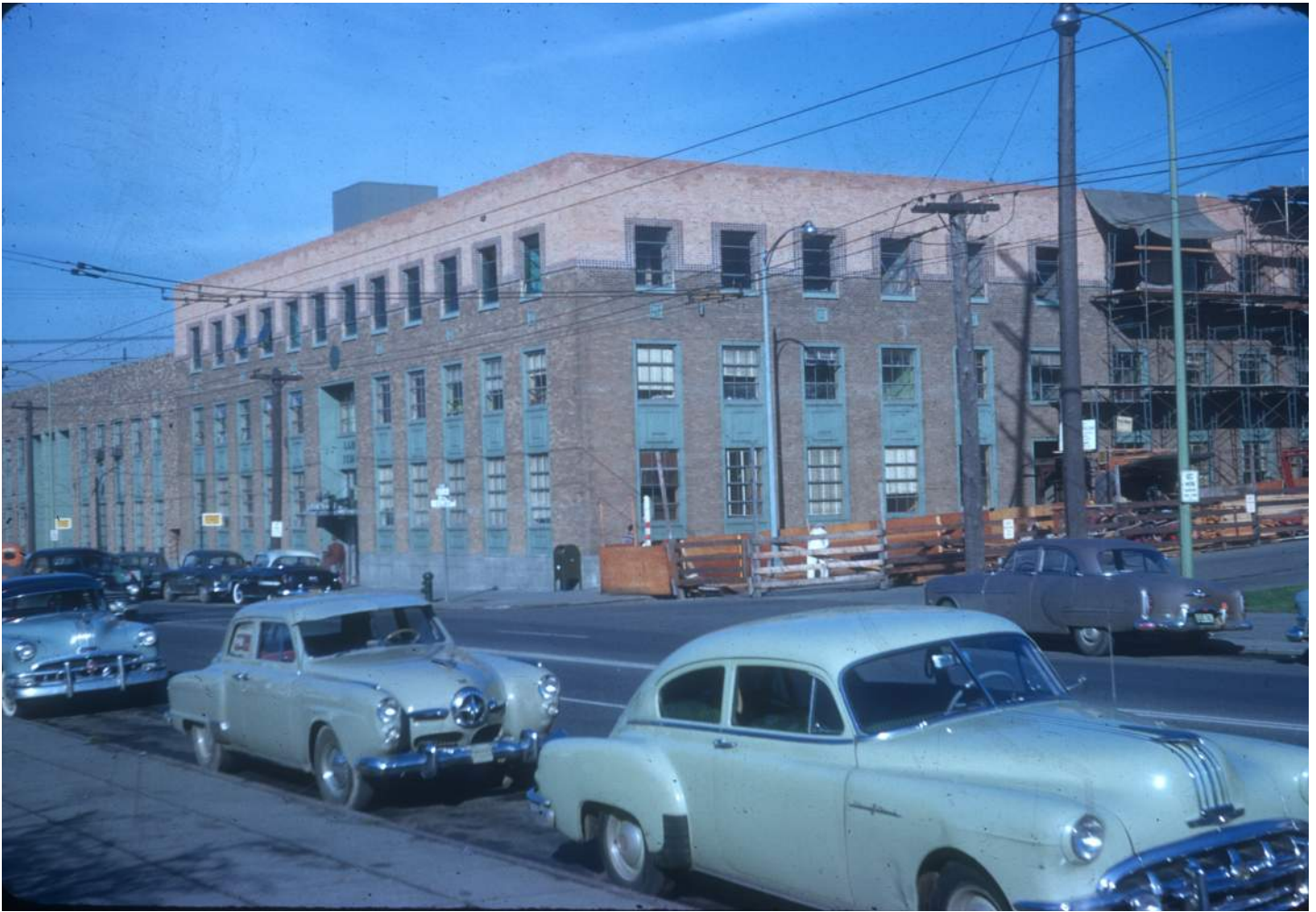
0.6 Kodachrome slide of Seattle Labor Temple, 2800 1st Avenue, taken by Reichert, c. 1955, with the annotation, “I did 3rd floor add’n.” The brick color of the new addition is clearly differentiated from the lower floors. The original building dates from 1942 and 1946, designed by McClelland and Jones; the addition is credited to Harmon, Pray and Dietrich, 1955. (UW College of Built Environments Visual Resources Collection).
