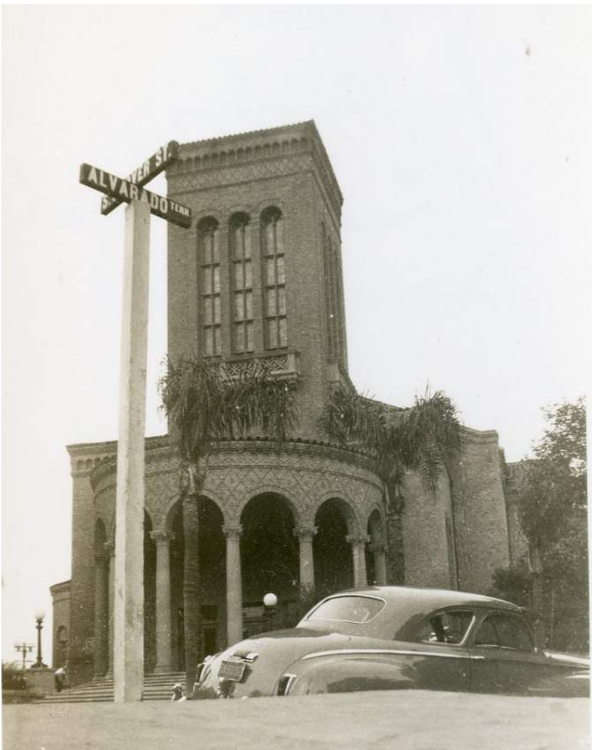
4.6 First Church of Christ, Scientist in Los Angeles (constructed 1912, designed by Elmer Grey), photograph by Robert Reichert. (Robert Reichert Collection, UW Libraries Special Collections UW39899).
