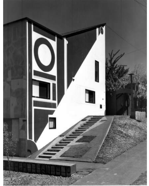
3.7 Reichert at the entry gate, c. 1957. Reichert at the house entry facing the garden. (Robert Reichert Collection, UW Libraries Special Collections UW39454).
