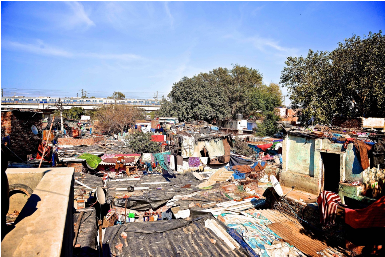
Figure 3.2. Picture showing the dense two-three storey dwellings at KPC, with Delhi Metro running in the background.
