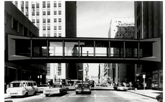
Figure 5 View of the first Minneapolis Skyway spanning over Marquette Avenue shortly after its construction in 1962.
