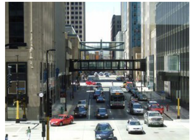
Figure 20 The Minneapolis Skyways ignore their surroundings, both the street and the buildings around it, making it a rather static and rigid infrastructure.
