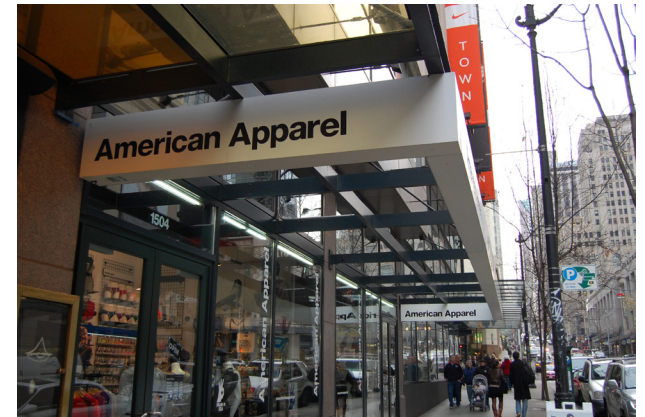
Figure 25 An example of overhead weather protection in Seattle, WA, it's part of the building code to include this on commercial buildings in the city.
