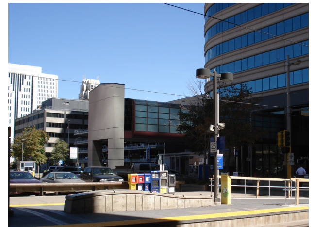
Figure 6 An example of a Minneapolis Skyway "dead-ending" where a potential new building could be built.
