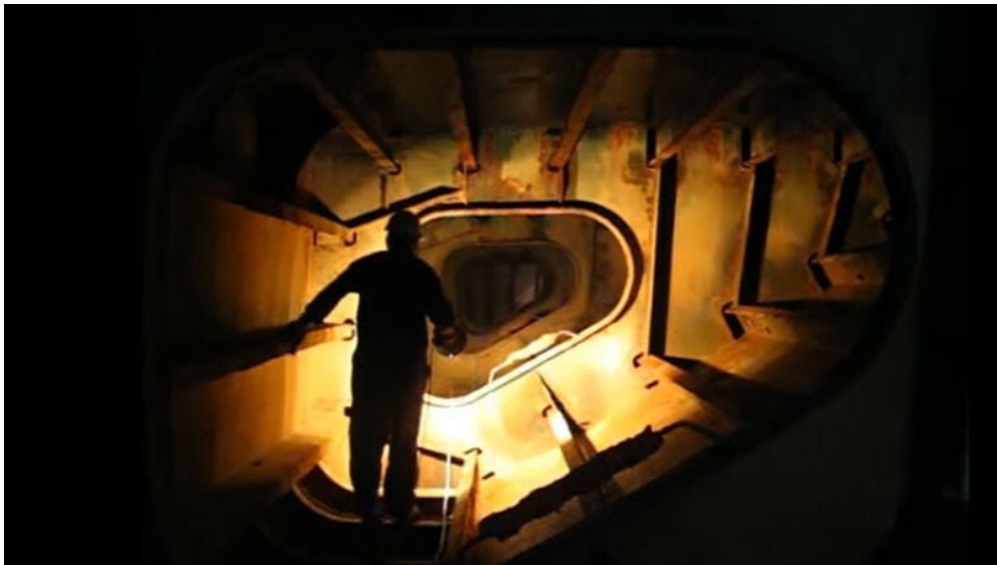
Figure 1.1: Example image of a worker inspecting a dry docked ballast tank 1
