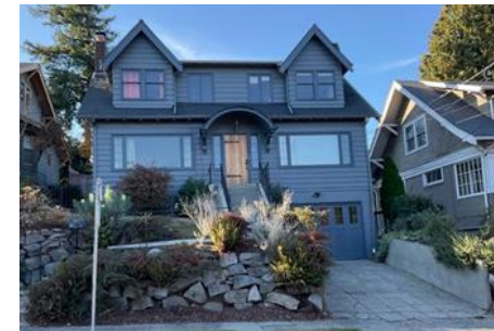
Figure #39. Duplex at 1927 25th Ave E (1928) in Current Single-Family Zone. by King County Assessor (public domain).
