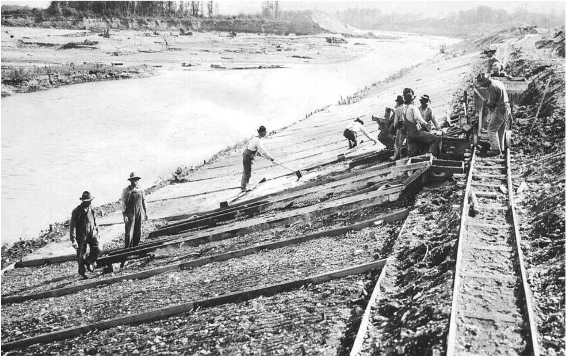
1915 – CONCRETE SIDE SLOPE
