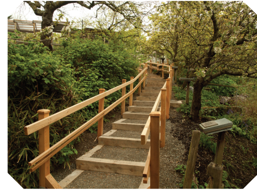
46' juniper, cedar & gravel staircase
