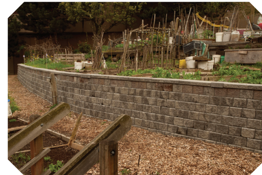
100' new block retaining wall
