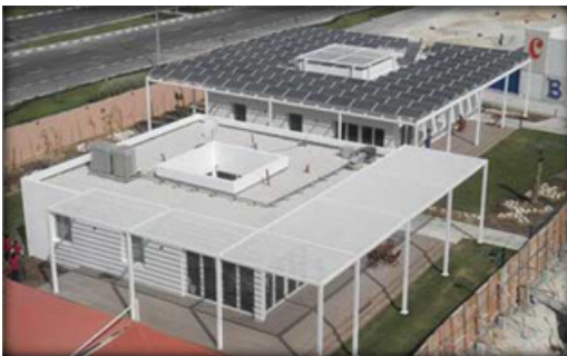
(Figure 3.1) The passive house Qatar next to the conventional house (source: (Khalfan & Sharples 2016))
