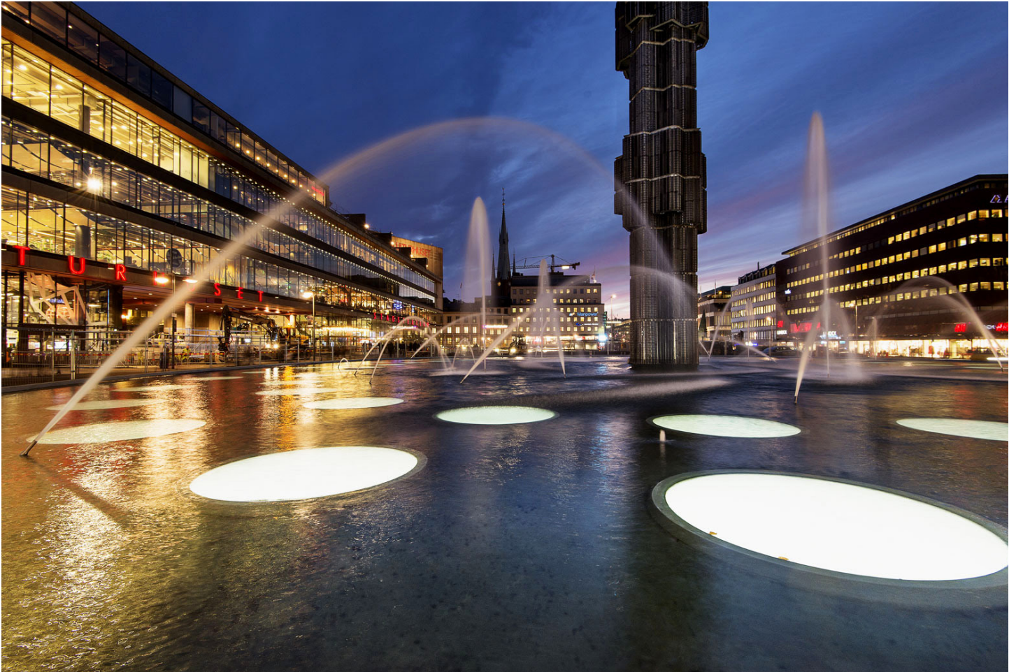
Figure 58 | The Fountain at Sergels Torg with Glazed Bottom Allowing a View from the Arcade Below. Copyright Heidelberg Cement Group.
