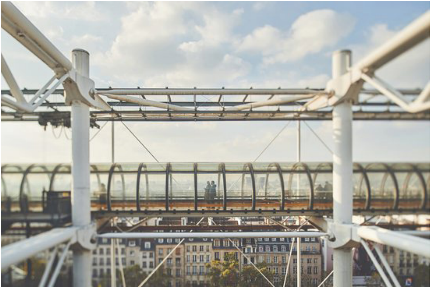
Figure 23 | View of Centre Pompidou Looking at External Circulation. © Manuel Braun 2015.
