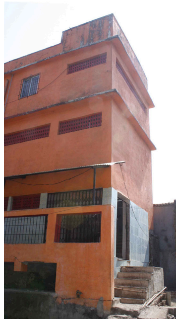
Image 36+37: Community Toilet Blocks
