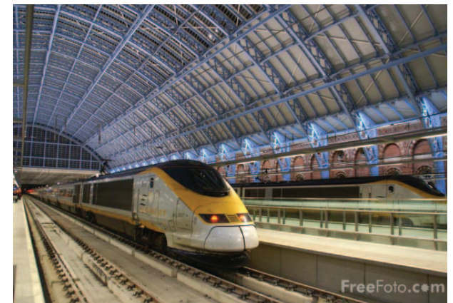
Figure 5.6 - View of tracks under glass and steel shed
