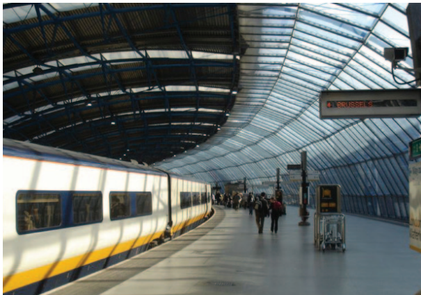
Figure 5.3 - Interior view of platform under barrel-vaulted roof
