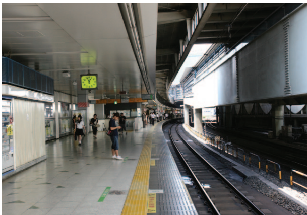
Figure 5.15 - Tracks in station during down time.
