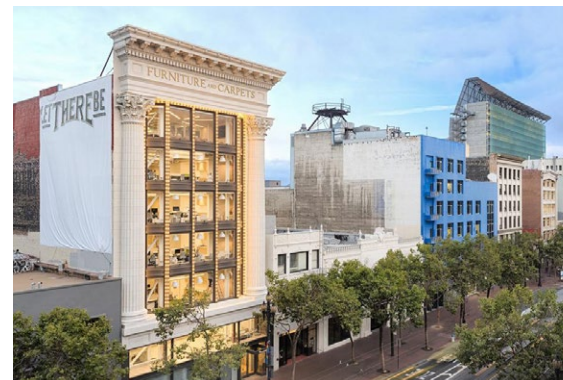
Figure 4-9: Zendesk in the historic Furniture and Carpets Building on Market Street
