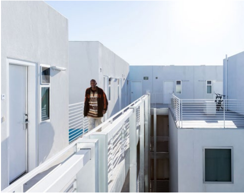
Figure 2-8: Exterior circulation, Star Apartments
