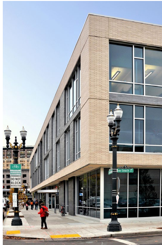
Figure A-9: Corner facade of OTRC
