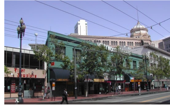
Figure A-13: The Hollywood Billiards building before its vacancy
