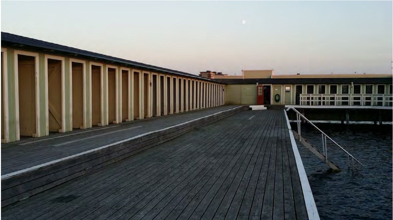
An extensive changing room and sun deck at Ribersborgs Kallbadhus. Image Source: Jesce Walz
