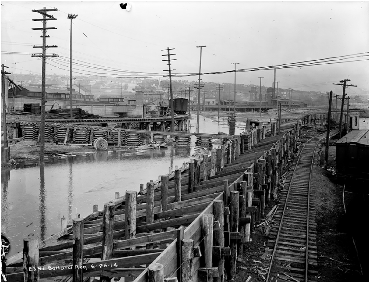
Fig. 2.21: Seattle Municipal Archives. Re-grading Shilshole Avenue to raise street above new water level, 1914
