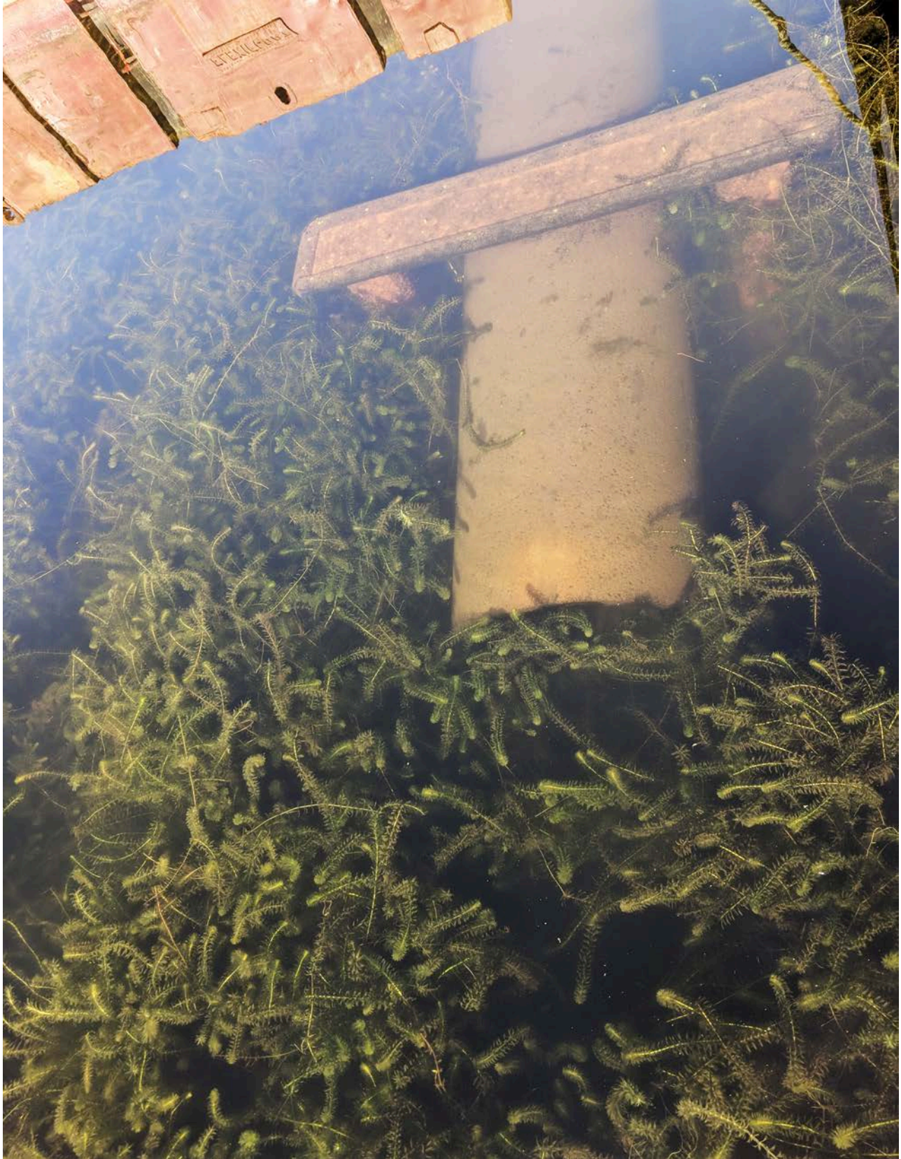
Fig 3.10: CSO # 150 at its outfall into Salmon Bay
