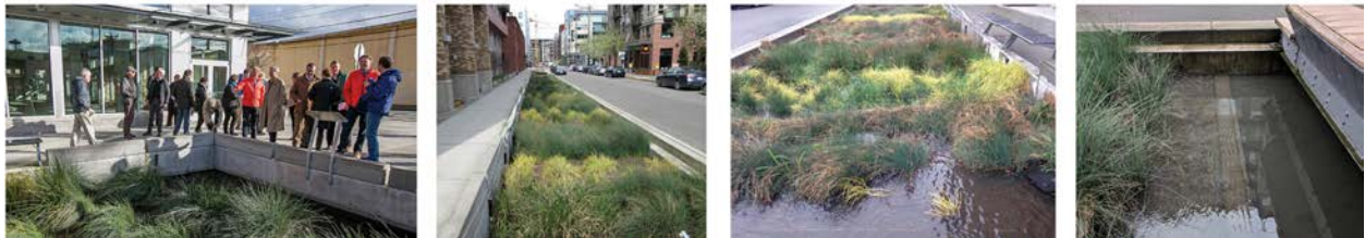
The Swale On Yale filters an average of 190 million gallons of stormwater each year (2013/2019)
