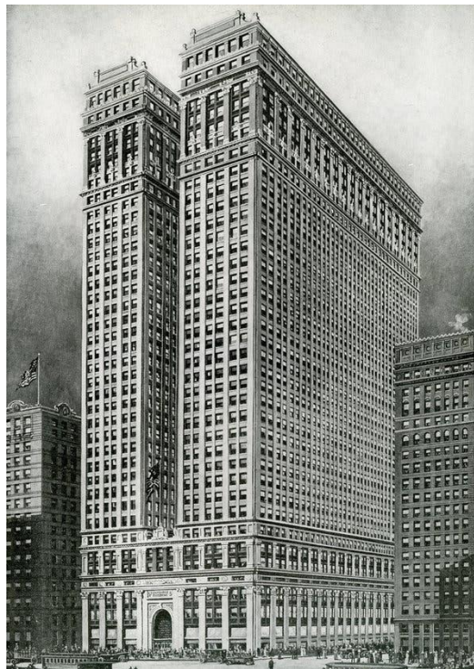
Figure 2. The Equitable Building. (King’s View of New York)
