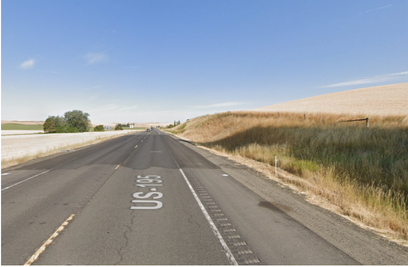
Figure 12 - 9914 US 195 Pre-Project Roadway View
