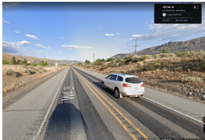
Figure 30 – XE3419 Pre-Project Roadway View
