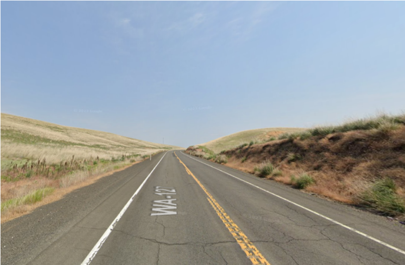
Figure 11 - 9914 SR 127 Pre-Project Roadway View
