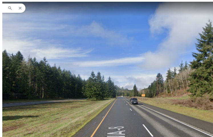
Figure 24 – XE3404 Pre-Project Roadway View
