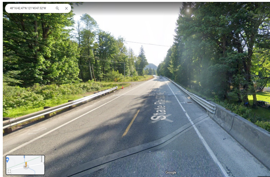
Figure 18 – 9954 Pre-Project Roadway View
