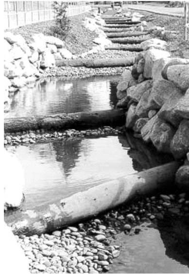
Seattle’s Viewland swale, a recent effort to increase stormwater infiltration.
