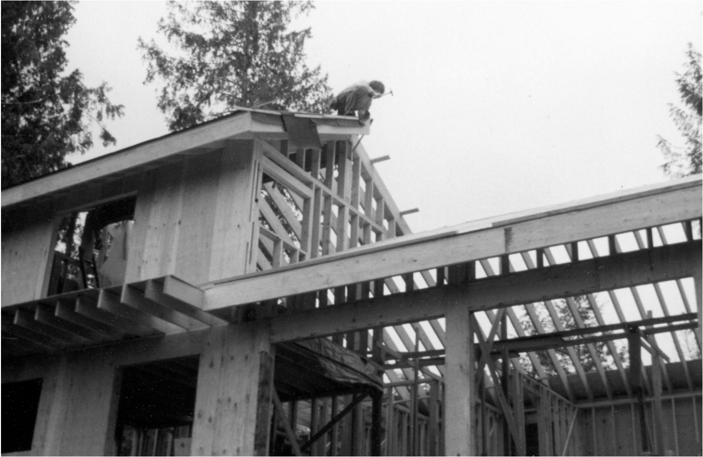
Fig 20. William Flintoff working on the roof of the house
