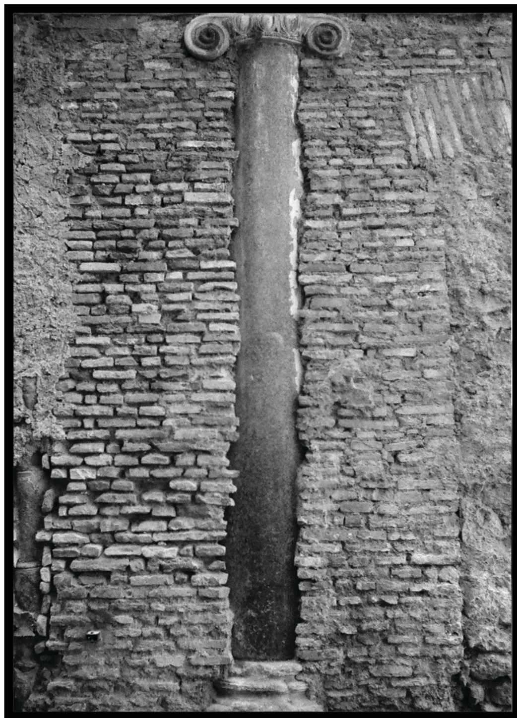
Fig 35. Ionic column between newer brick construction. Rome, Italy (photograph by author)
