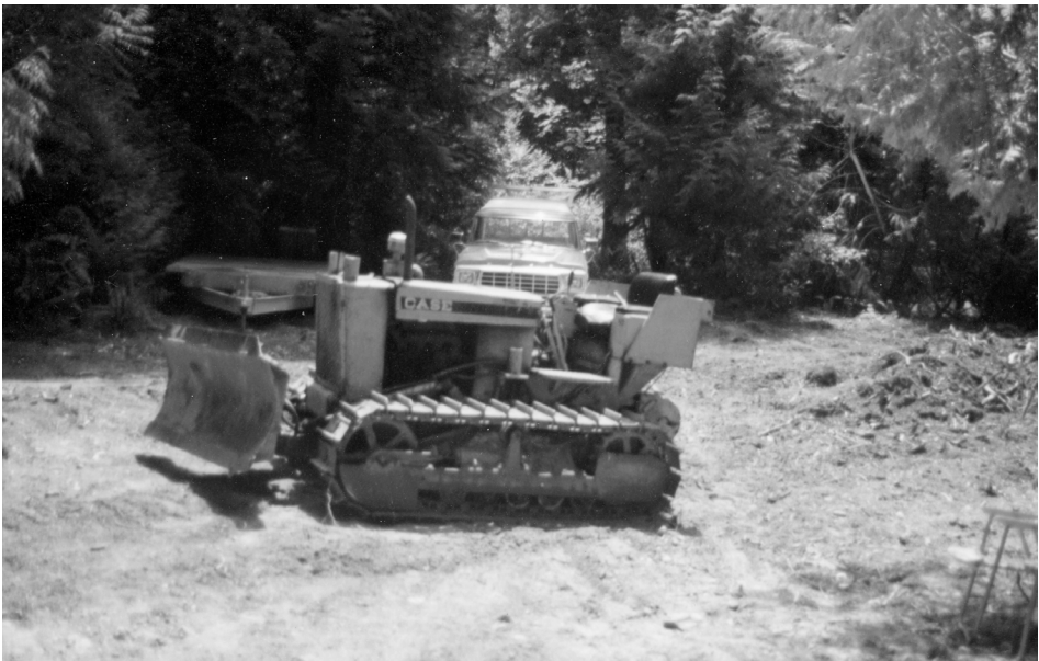
Fig 18. Williams bulldozer for clearing land
