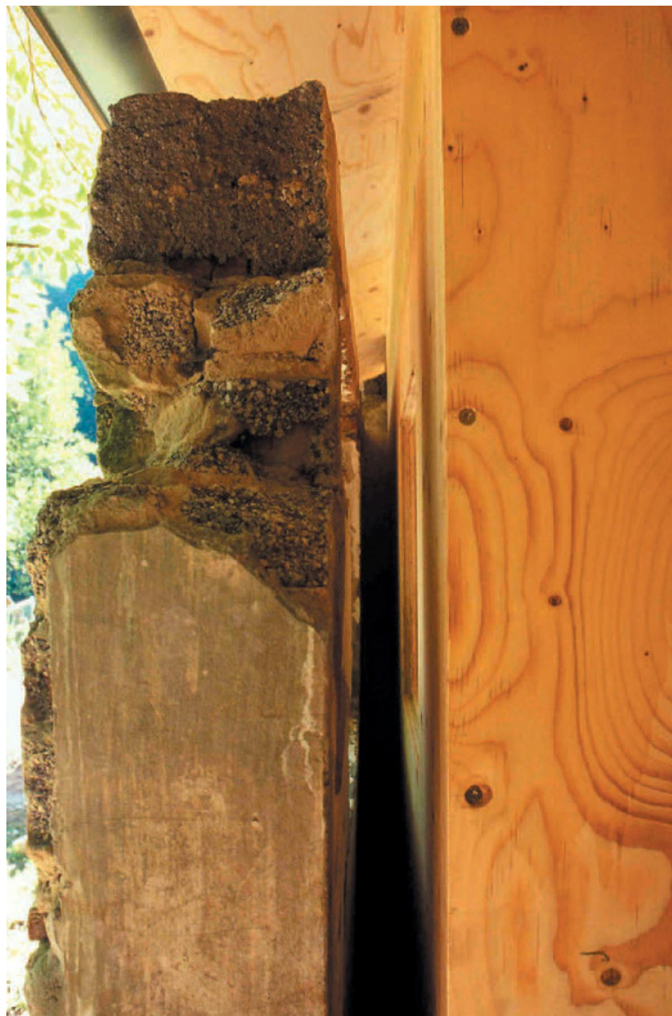
Fig 68-69. Naumann Architektur Showroom (photographer Zooey Braun https://www.subtilitas.site/ post/101190397924/naumann-architektur- renovation-of-a-dilapidated )
