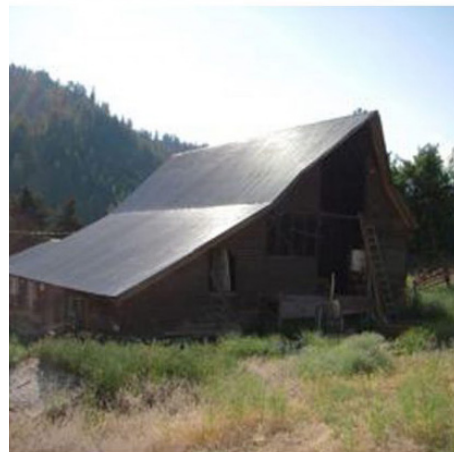
Fig 55-60. Finished photos and drawings of MWworks Canyon Barn (photographs by Tim Bies)
