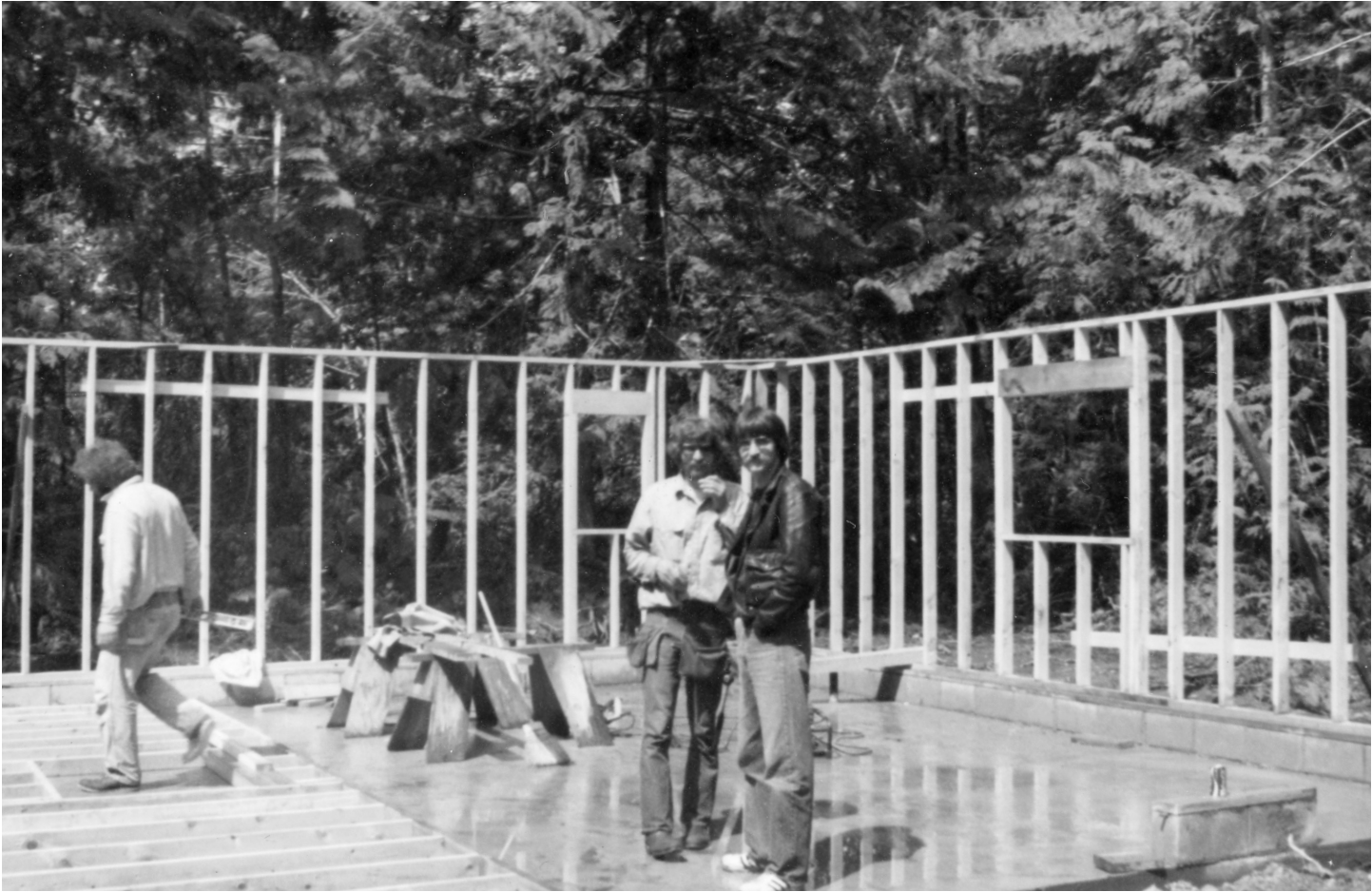
Fig 19. William Flintoff and brothers framing the garage
