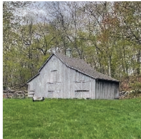
Fig 49-51. 1980s Horse Barn to Studio Barn (Photographs by Naho Kabota, https://www.worellyeung.com/home/studio-barn )
