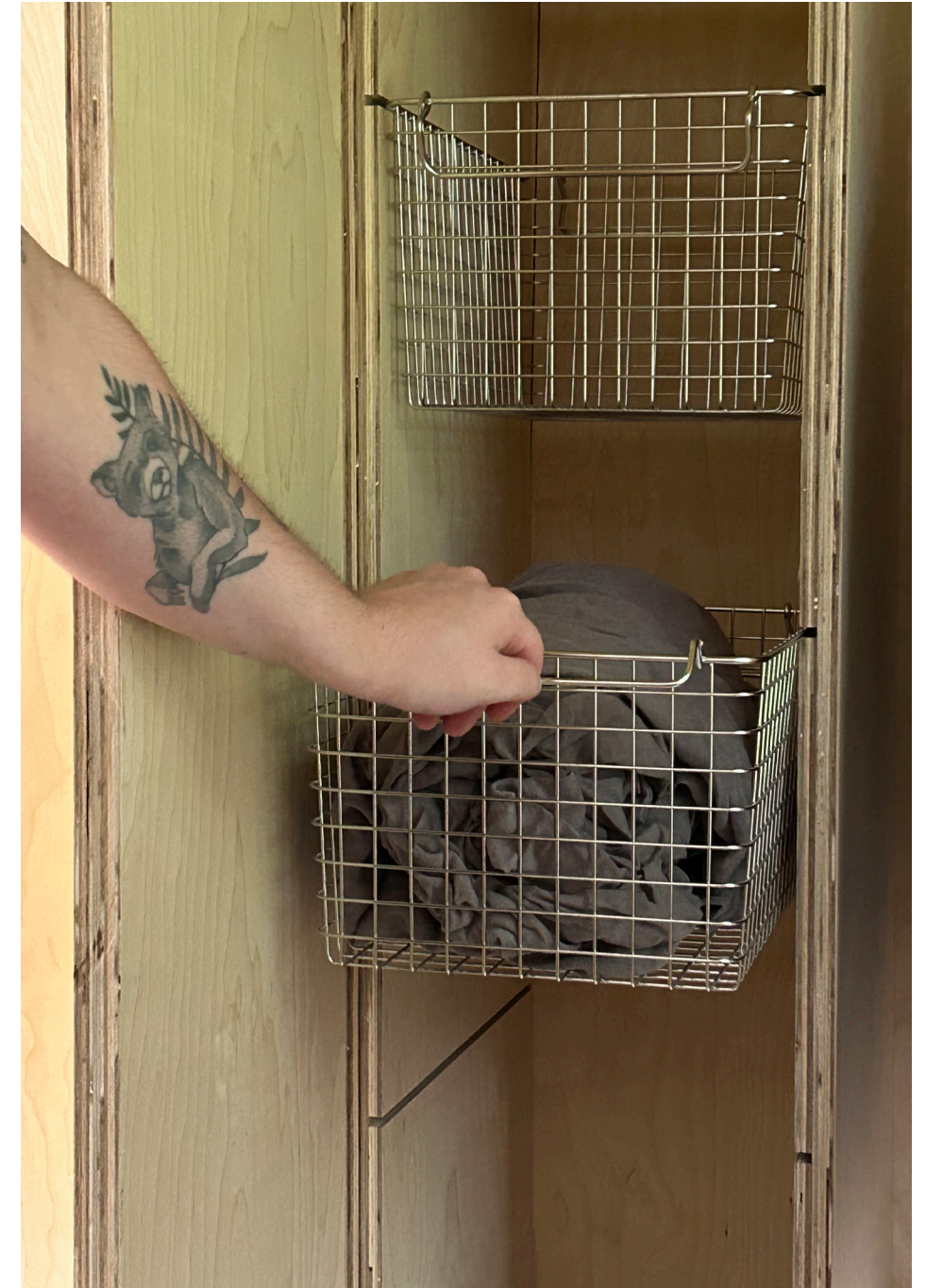
The closet incorporates a friction-fit basket drawer system assembled through routed dado's, allowing storage to remain flexible and integrated within the built-in closet system.
