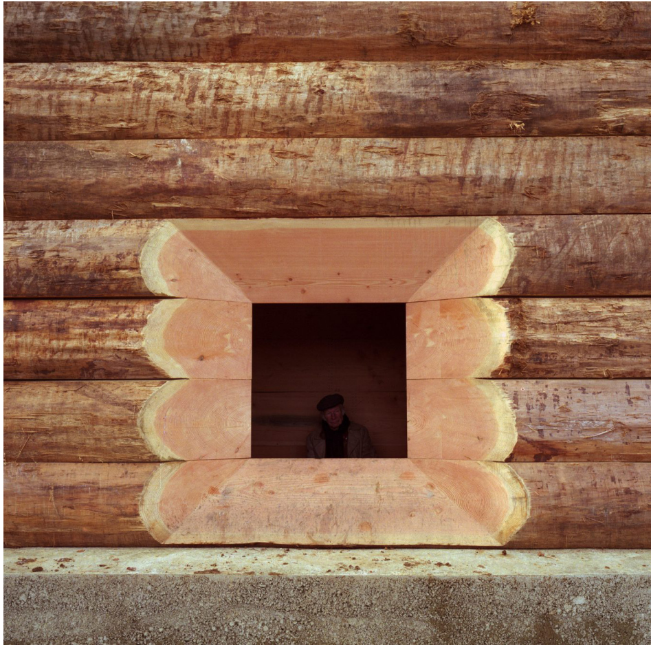
Fig 44-45. John Pawson's wooden chapel, built from carving 61 stacked logs in Unterliezheim, Germany. (photographer Eckhart Matthäus)
