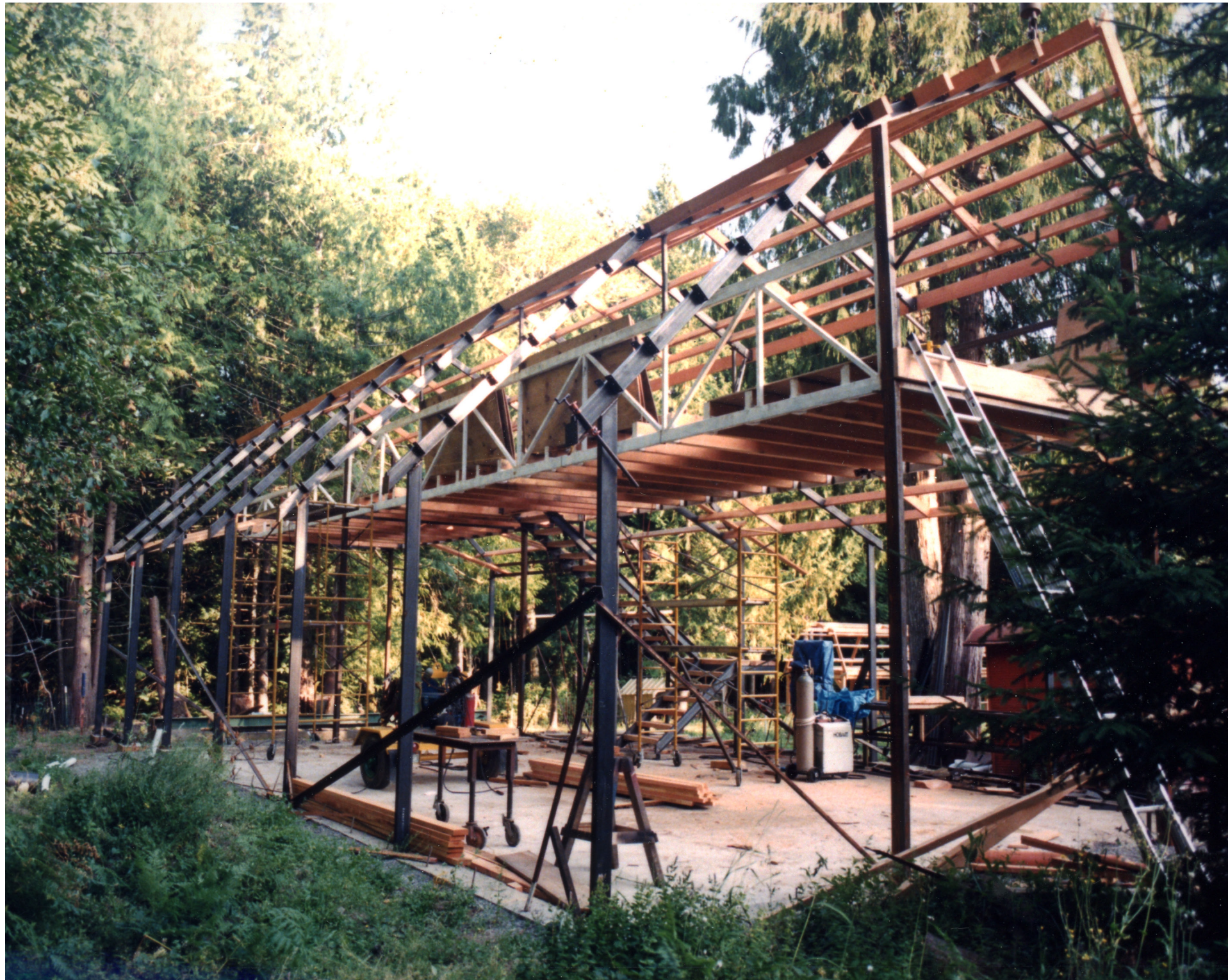
Fig 21-22. Big barn under construction 1995. Photographs by William Flintoff
