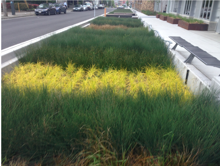
Figure 64. The Swale on Yale is an $11M biofiltration system in South Lake Union that will consist of four biofiltration swales, a pre-treatment swirl concentrator, a diversion vault, and 2000ft of new storm drain when completed. Two swales were completed in 2013, and two more will be constructed 2017-2018 after two years of monitoring and possible design modifications. The system will treat an average of 190 million gallons of runoff from 630 acres annually in one of the most densely urbanized areas of the city. Each swale is 270-feet long by 10.5 to 16.5-feet wide. The diversion vault is a large underground tank that diverts the stormwater into the biofiltration swales. The swirl concentrator spins the stormwater to create a vortex, which separates large solids and trash into a sump that has to be cleaned regularly. 112 Image source: author.
