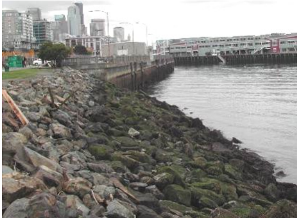
Figure 18. OSP shoreline before restoration.
