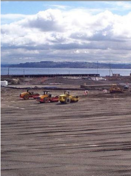
Asarco smelter site after being razed and capped. Image from US Environmental Protection Agency.
