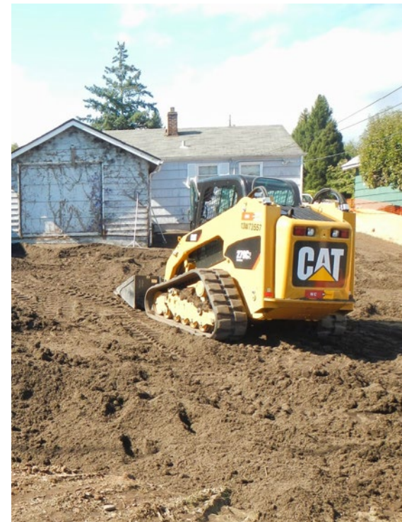
Residential yard receiving new, clean backfill after excavation of contaminated soils. Image from Washington State Department of Ecology.
