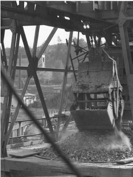
Ore being fed through Tacoma smelter. Image from Tacoma Public Library.
