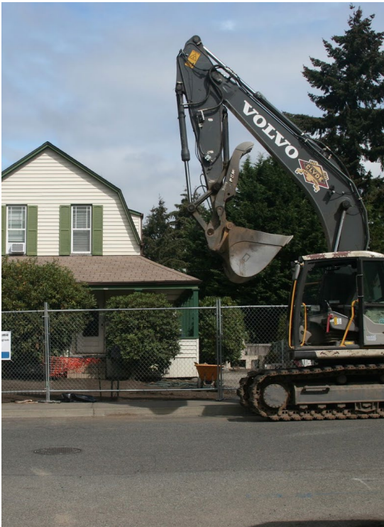
Excavator poised to remove contaminated soils from front yard. Image from Washington State Department of Ecology.
