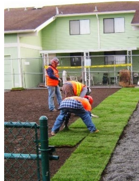
Yard receiving new sod after toxic soils excavated from Everett smelter contamination. Image from Washington State Department of Ecology.
