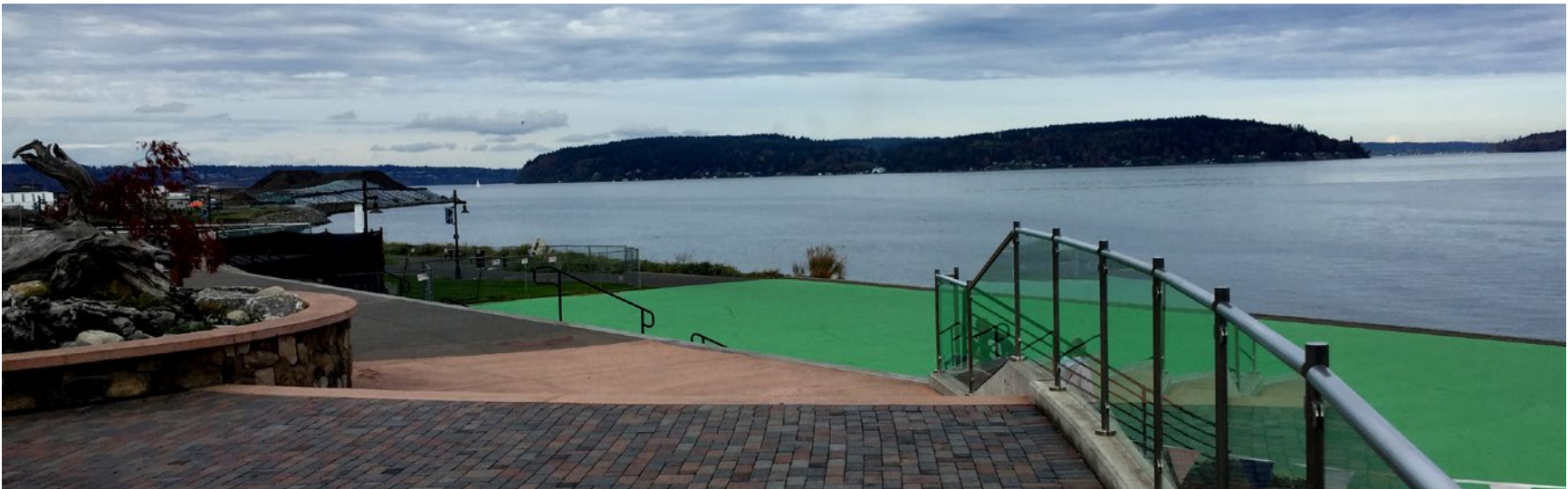
View of freshly painted plaza on Point Ruston waterfront. Author's image.
