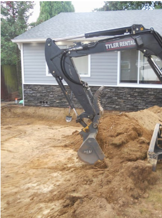
Residential yard in Ruston in process of excavating contaminated soils. Image from Washington State Department of Ecology.
