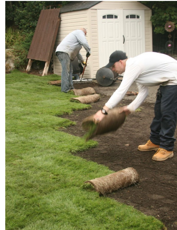
Sod being laid in a remediated yard in Ruston, WA. Image from Washington State Department of Ecology.
