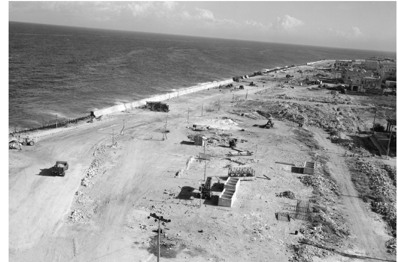
Figure 07: El Malecón under construction
