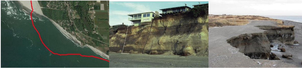
Figure 1-1: Coastal erosion threatening roads and coastal infrastructure. Left) Washaway Beach in Washington, red line was shoreline in 1990, image is from 2017. Middle) Gleneden beach in Oregon, example of cliff erosion that could also influence coastal roadways. Right) Port Heiden in Alaska was disconnected because of road failure in 2017.
