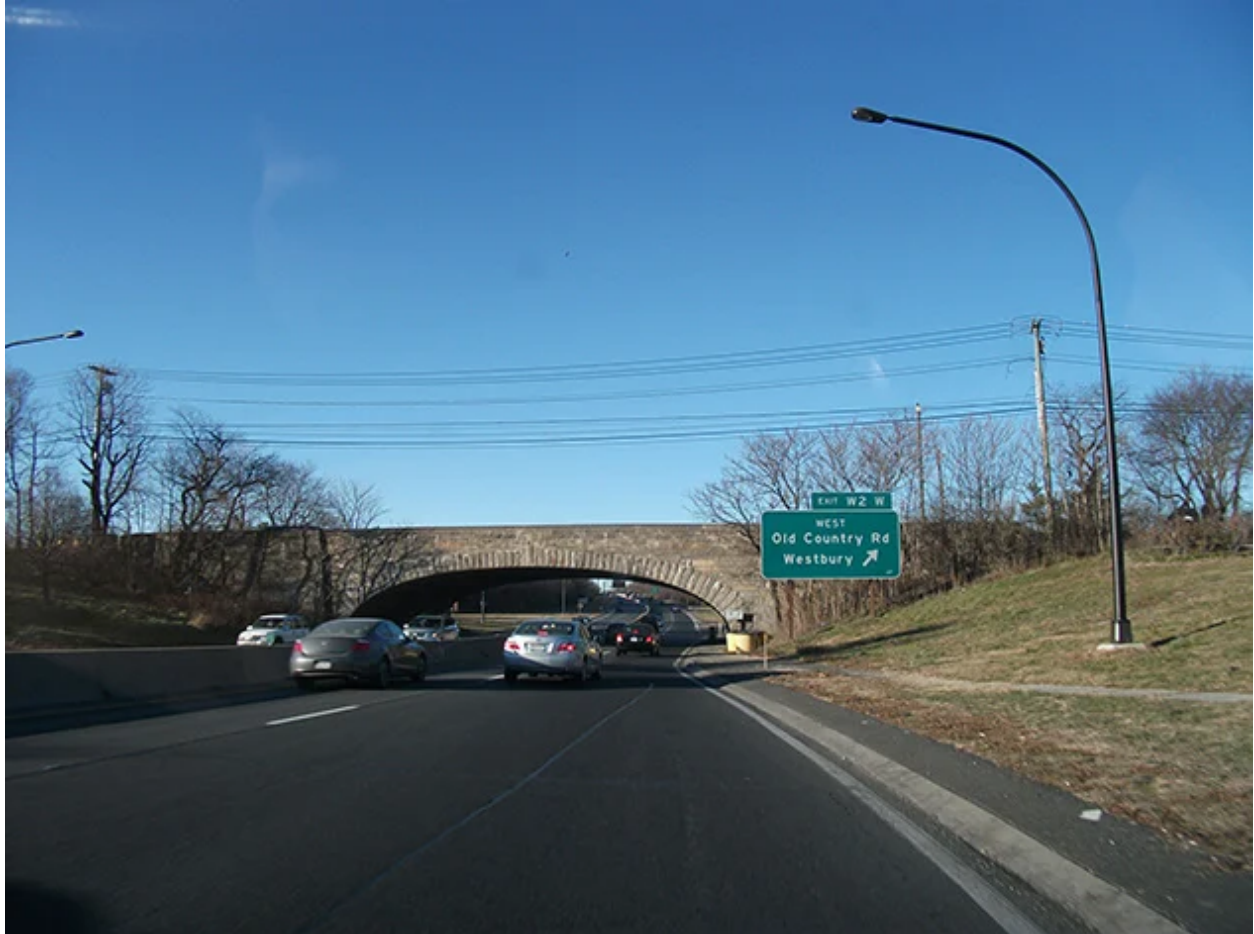
Figure 1: Low overpasses on a Long Island freeway. Source: Doug Kerr via Flickr
