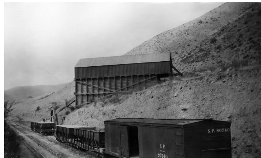
50 Lower terminal and dump shoot of aerial tramway.
