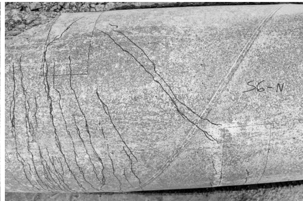
f) Specimen 6 north span concrete cracking
