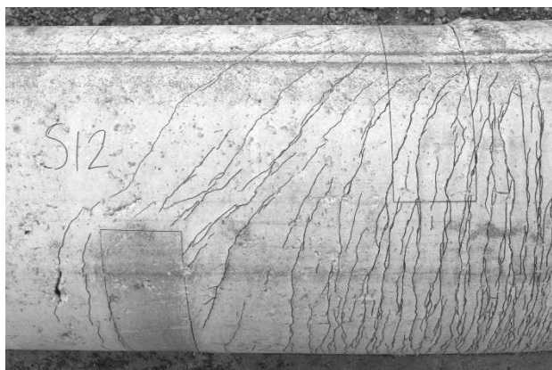
e) Specimen 12 north span concrete cracking
