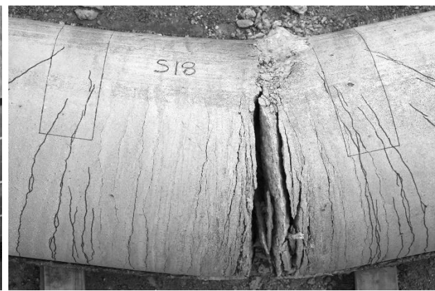
d) Specimen 18 mid-span concrete cracking
