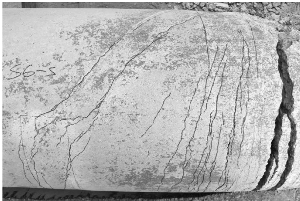
e) Specimen 6 south span concrete cracking
