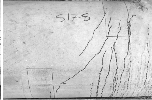
Figure 5.3: Minimal shear cracking
