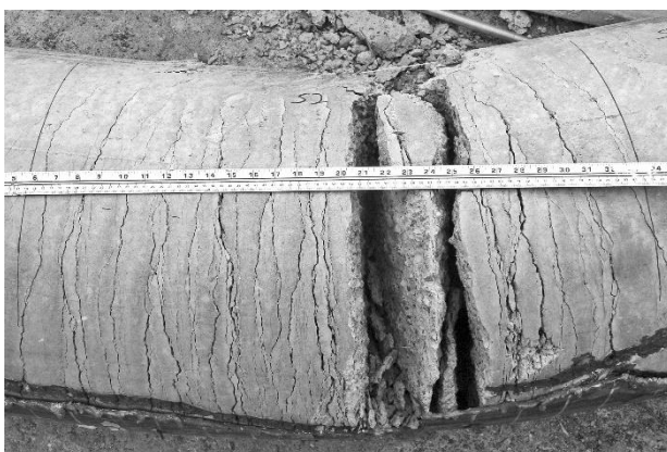
d) Specimen 2 mid-span concrete cracking
