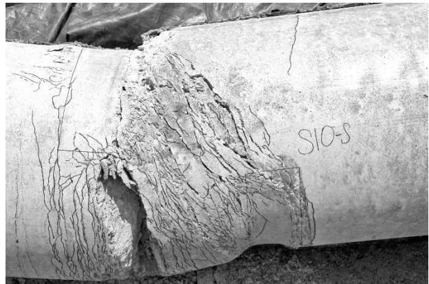
f) Specimen 10 south span concrete cracking
