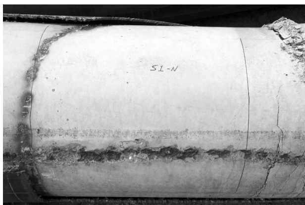
e) Specimen 1 north span concrete cracking
