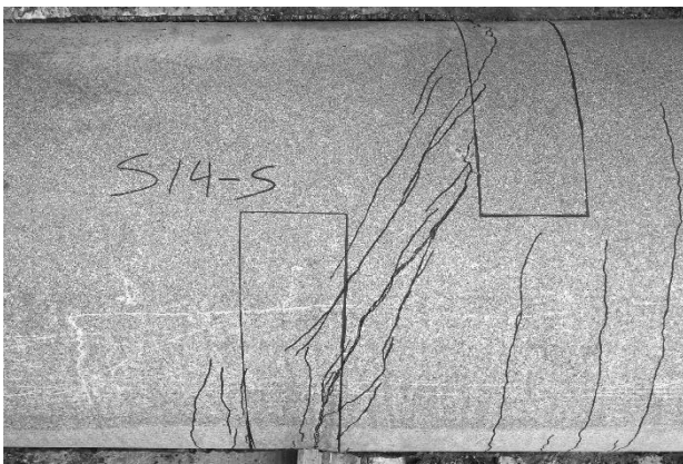
e) Specimen 14 south span concrete cracking
