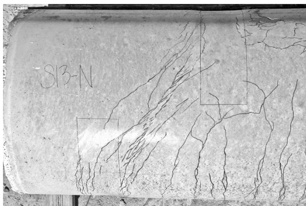
e) Specimen 13 north span concrete cracking
