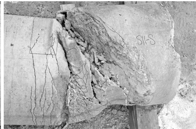
f) Specimen 11 south span concrete cracking
