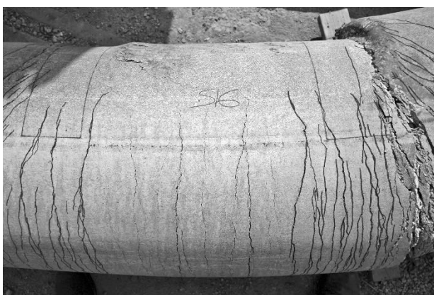
d) Specimen 16 mid-span concrete cracking
