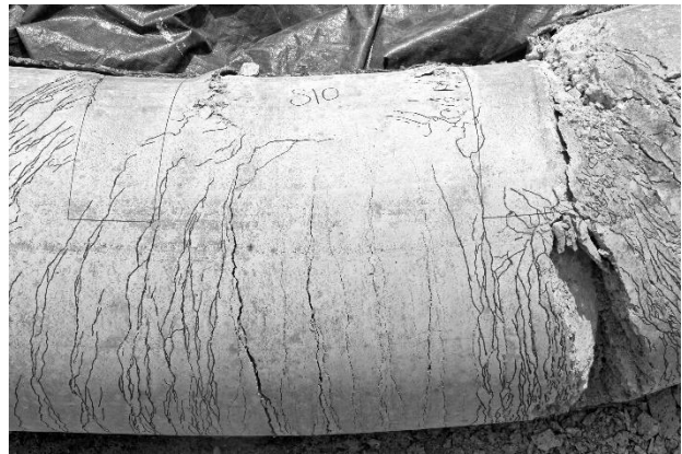
d) Specimen 10 mid-span concrete cracking
