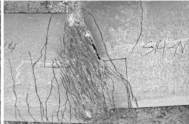
Figure 5.7: Extensive shear cracking
