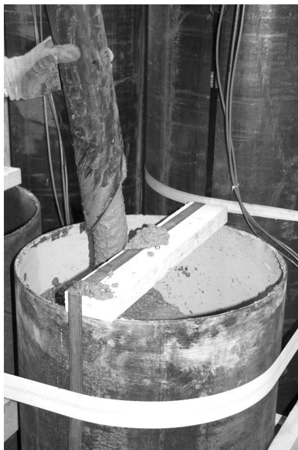
Figure 3.19: Concrete pumping
