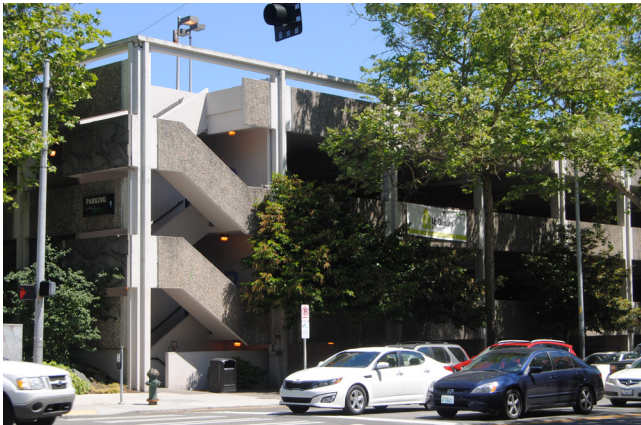
Figure 2: Mercer Street Parking Garage: Regularity of Structural Ordering; Source: O'Lone, Katie. Mercer St. Parking Garage . Photograph. Seattle, WA: June 7, 2015.
