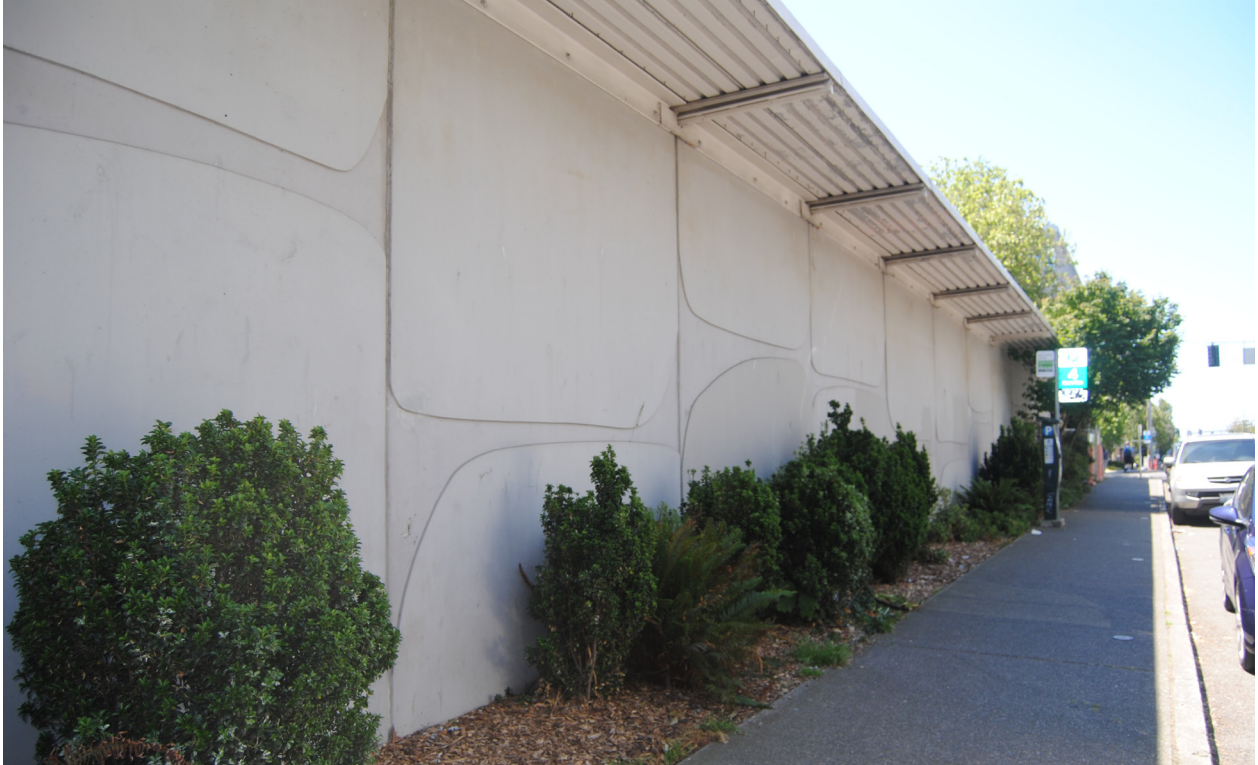
Figure 35: Northwest Rooms - North Side of Building; Source: O'Lone, Katie. Northwest Rooms - N. Side . Photograph. Seattle, WA: June 7, 2015.
