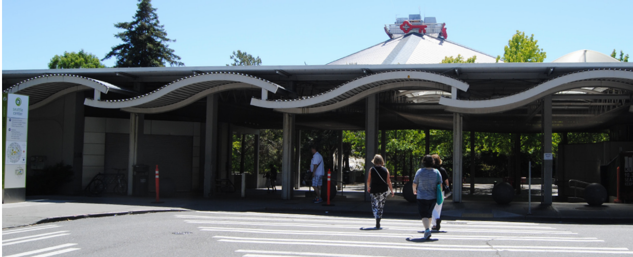
Figure 36: Northwest Rooms - Awning and Break in Building; Source: O'Lone, Katie. Northwest Rooms - N. Side . Photograph. Seattle, WA: June 7, 2015.
