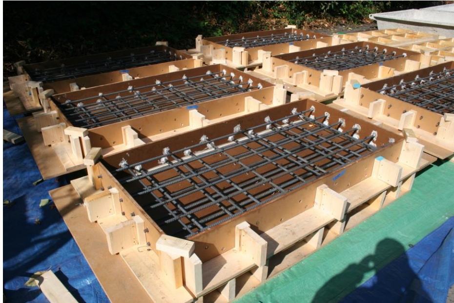
Figure A.8: Bridge Deck Slab Formwork Placed Outside Awaiting Ready-Mixture Truck
