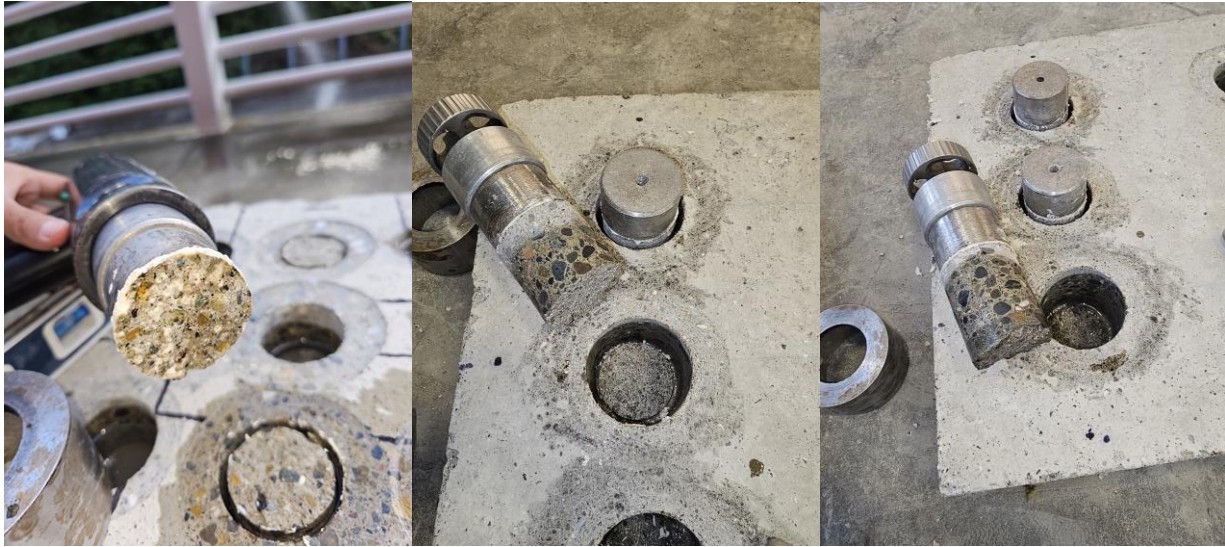
Figure 5.8: Typical Bond Test Failure Types
