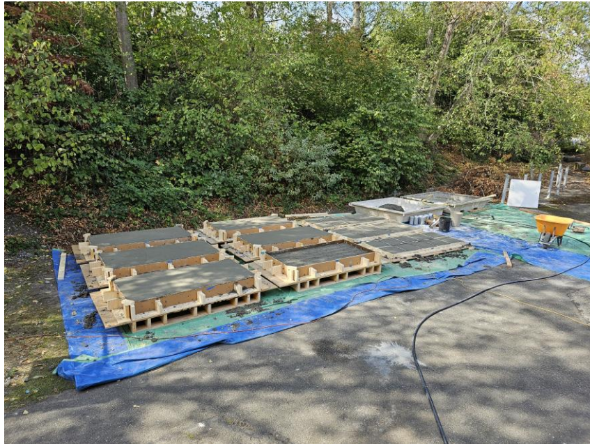
Figure 3.7: Concrete Pour Finished
