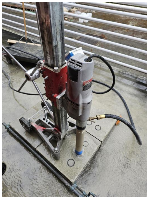
Figure 3.26: Concrete Coring for Bond Testing
