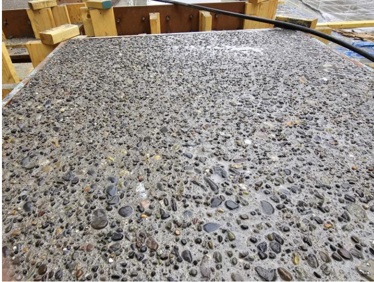
Figure 3.9: Exposed Aggregate Etching
