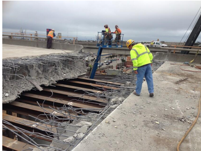
Figure 1.2: Hinge Replacement on I-208 Freeway from [21]
