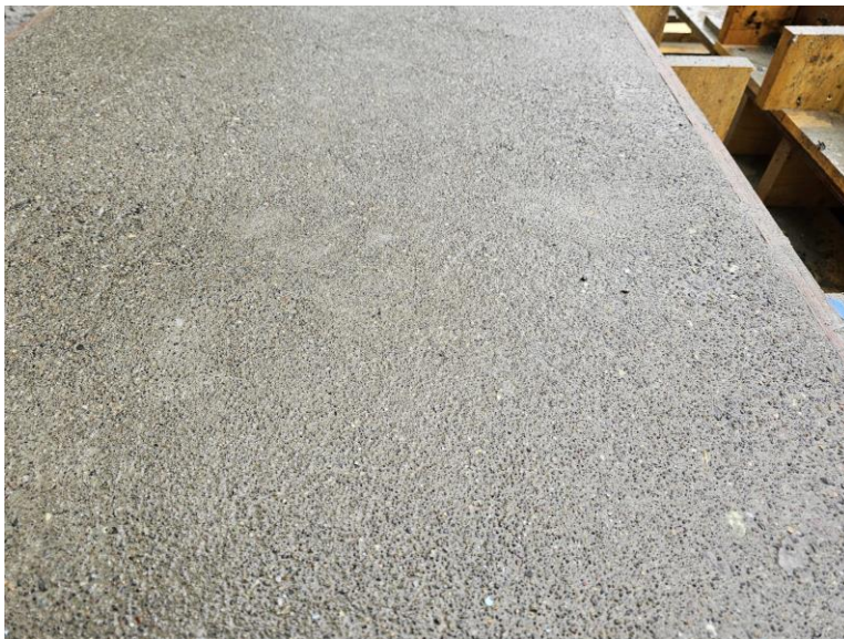
Figure 3.10: Sandblast Etching
