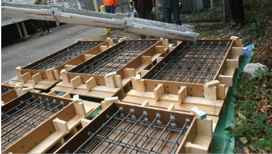
Figure A.9: Read-Mixture Truck Before Pouring with Chutes Attached
