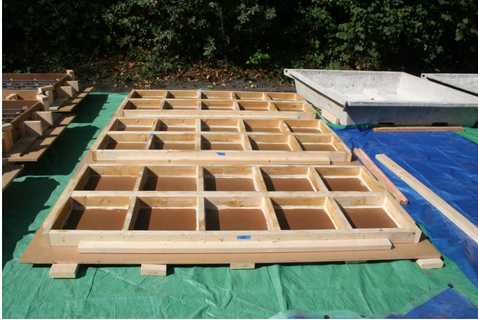
Figure A.7: Paver-Sized Substrate Formwork Placed Outside Awaiting Ready-Mixture Truck
