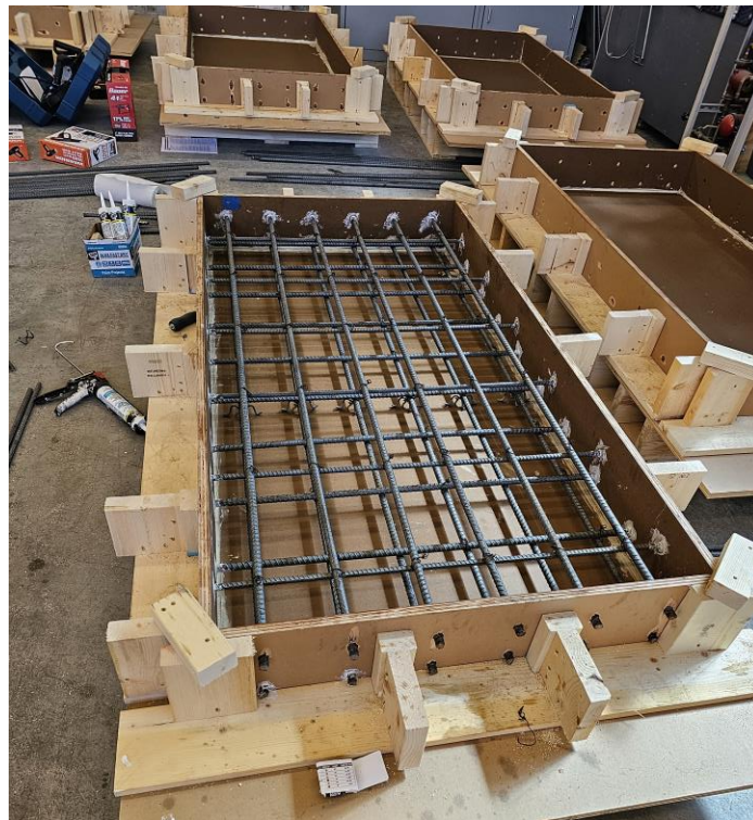
Figure A.5: Bridge Deck Slab Formwork.
