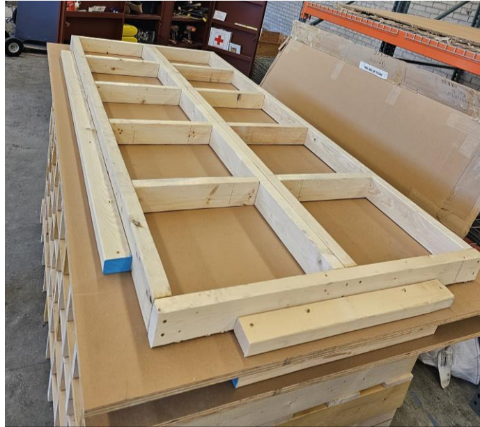
Figure A.6: Paver-Sized Substrate Formwork.
