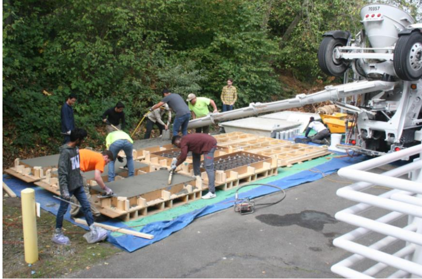
Figure 3.6: Concrete Cast in Progress
