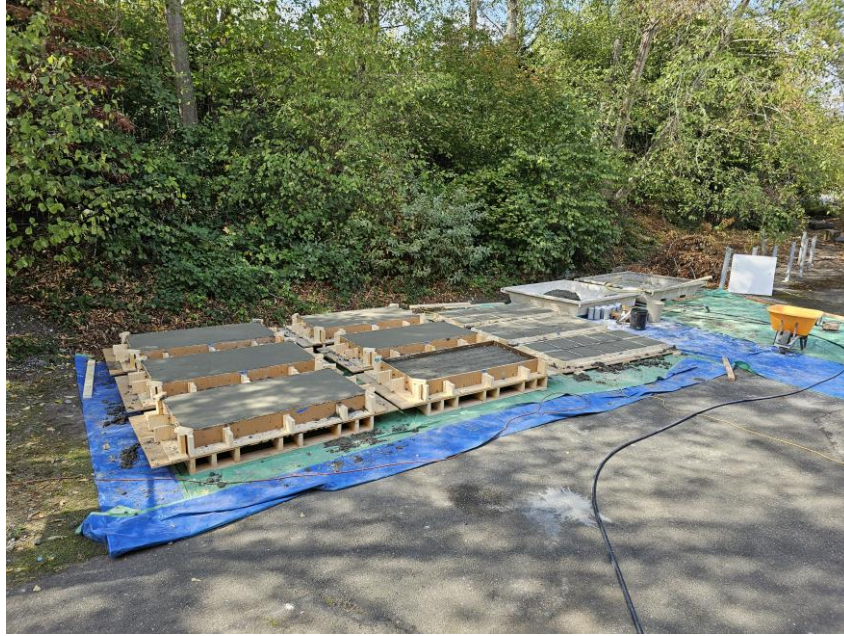
Figure A.11: Concrete Pour Finished
