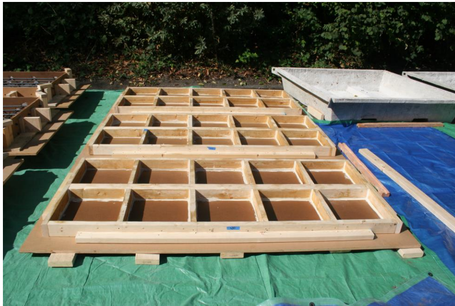
Figure 3.5: Paver-Sized Substrate Formwork Placed Outside Awaiting Ready-Mix Truck
