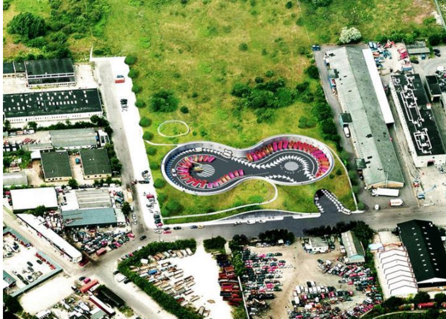
Figure 18 Sydhavyns Recycling Center from BIG
