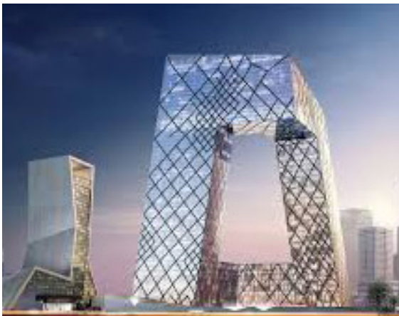
Figure 6. OMA. Beijing CCTV Headquarters in Beijing
