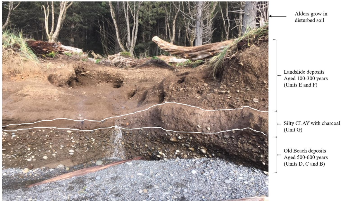
Figure 26. Marine terrace exposure on October 23, 2019, showing landslide debris dated to ~300 years calBP overlying aquitard clay layer, which caused multiple seeps along the terrace face. Below this is Old beach, dated to be between 500-600 years calBP.
