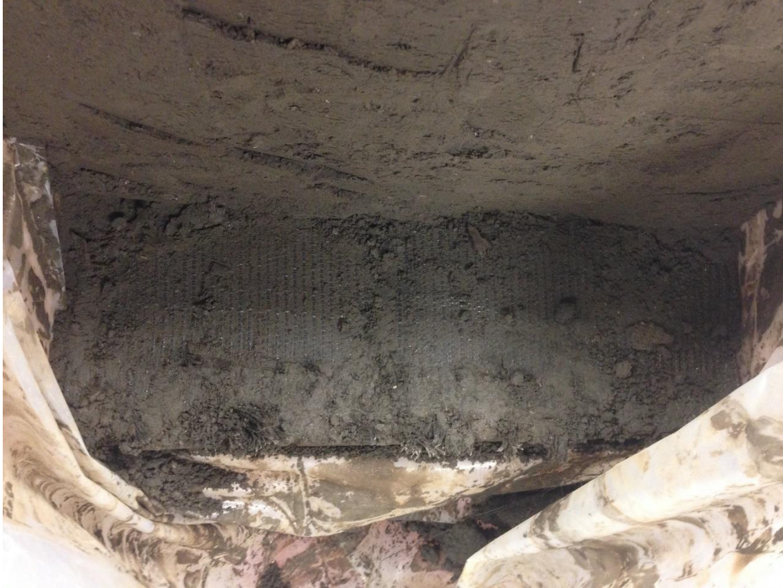
Figure 4.6 Photo of organic silt and blinding of the fabric at the bottom.
