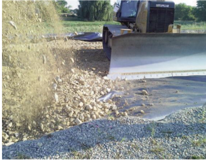
Figure 2.20 Field Construction at Jefferson County, WI
