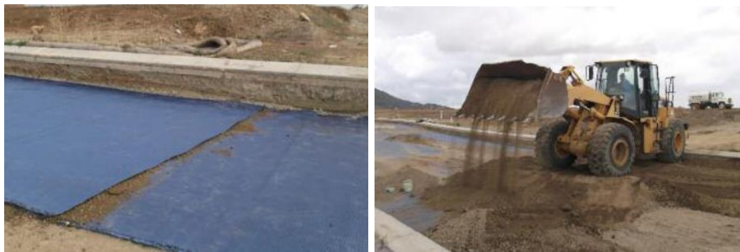
Figure 2.19 Field Construction at Corona, CA
