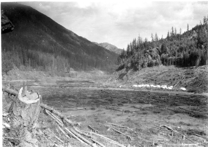
Fig. 44 Lake Mills logged for inundation photograph courtesy Clallam County Historical Society
