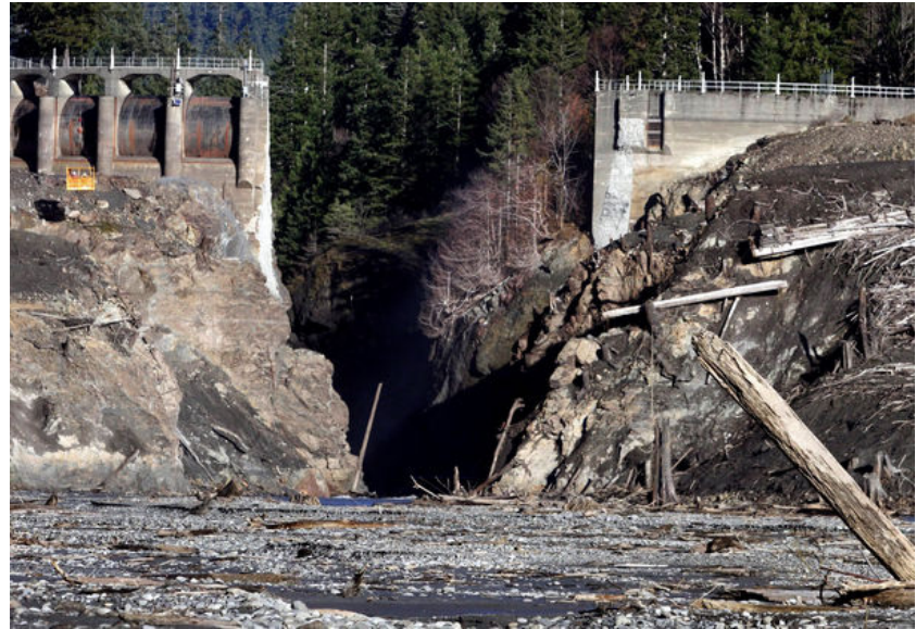
Fig. 29 Glines Canyon Dam mostly removed photograph by Greg Gilbert March 16, 2013
