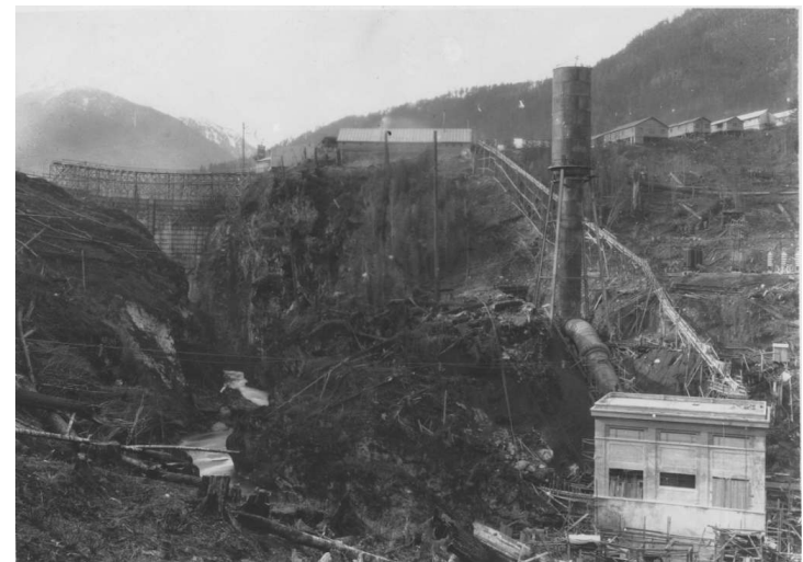
Fig. 24 Glines powerhouse under construction photograph by Robert Clawson
