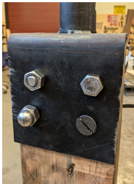
Figure 29. Fastener Choices for Column Cap and Stirrup. Upper left: hex nuts on both sides with a threaded rod in the middle. upper right: hex bolt with a hex nut on the other side. lower left: hex cap nuts on both sides with thread rod. lower right: flat head Slotted/Phillips machine screws with a hex nut on the other side.
