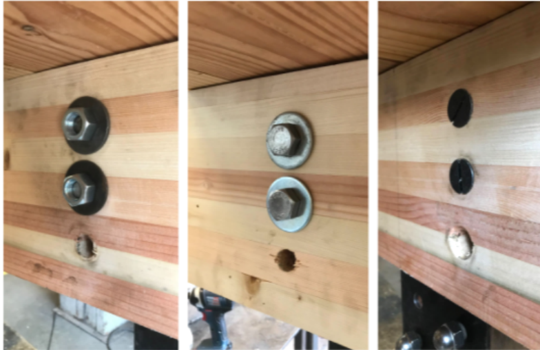
Figure 28. Fastener Choices for Glulam Beams. (from left to right): hex nuts, threaded rod with washers; hex tap bolt with washers or serrated hex flange screws; flat head Slotted/Phillips machine screws
