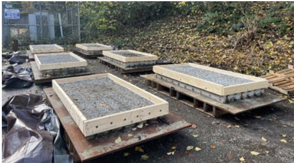
Figure 3-13: Completed formworks for all overlays
