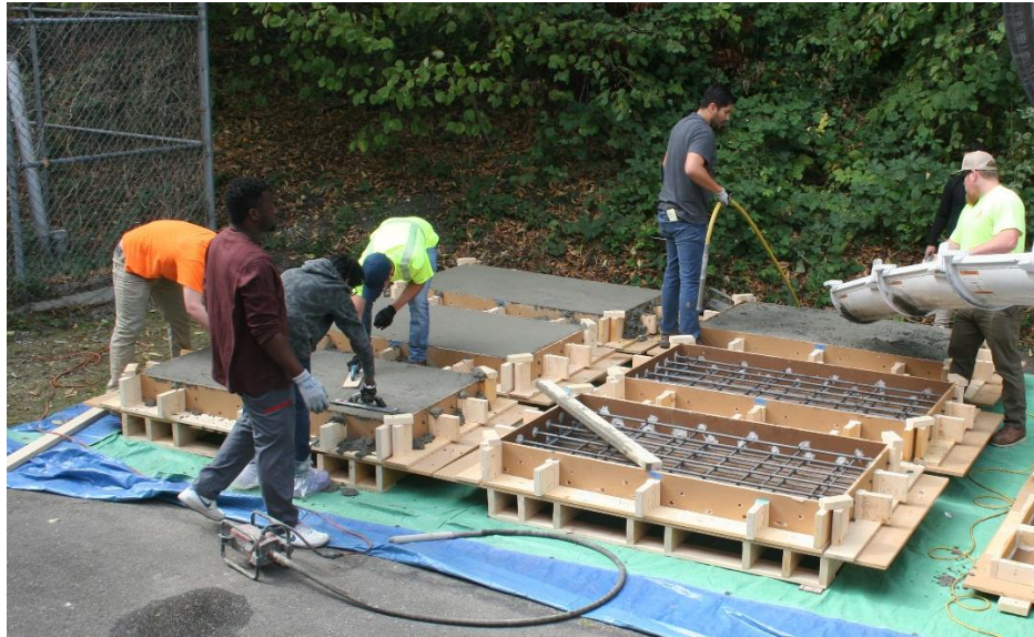
Figure 3-6: The substrate decks during casting (Guerrero-Estrada, 2024)
