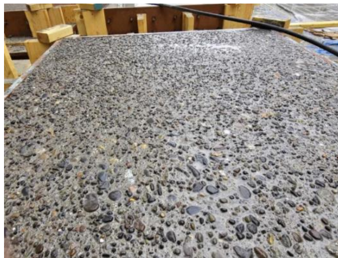
Figure 3-8: Exposed aggregate etching (Guerrero-Estrada, 2024)
