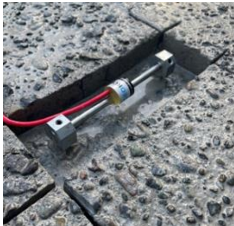
Figure 3-17: Close-up of an arc-welded strain gauge installation
