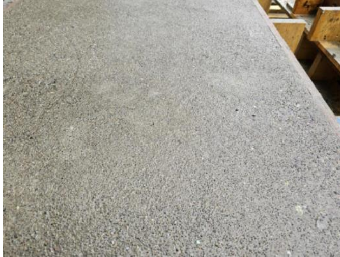
Figure 3-9: Sandblast etching (Guerrero-Estrada, 2024)
