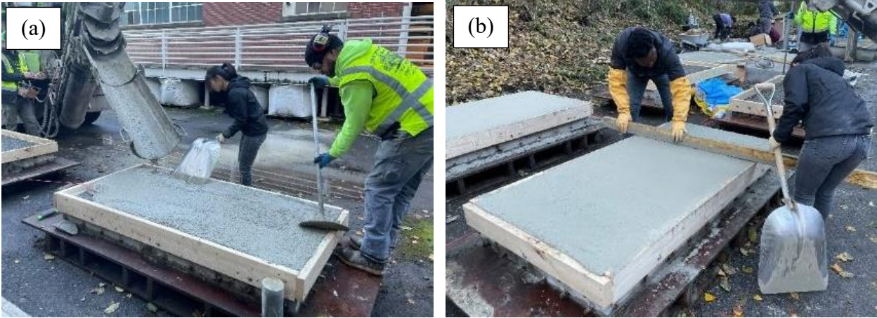
Figure 3-19: Casting (a) and screeding (b) of the mini-bridge deck overlays
