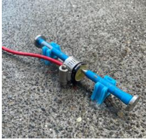
Figure 3-16: Close-up of a concrete-embedded strain gauge installation
