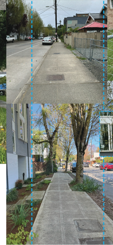
SIDEWALK CONDITION ALONG CLOVERDALE IS VARIABLE WITH MINIMAL TO NO BUFFER
