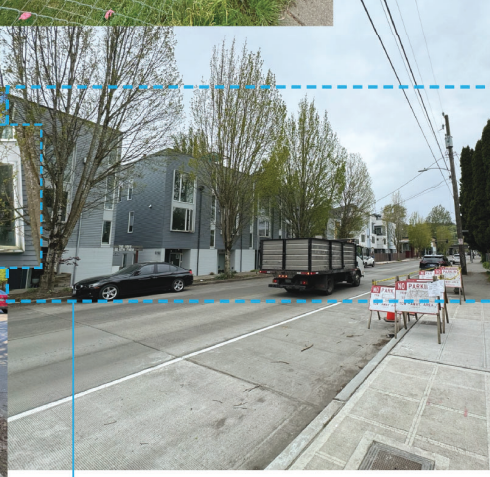
HIGHER DENSITY DEVELOPMENT WITH LONG SPANS OF MONOLITHIC FACADES CREATE URBAN CANYONS
