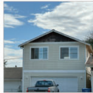
COMPROMISED INDOOR AIR QUALITY
