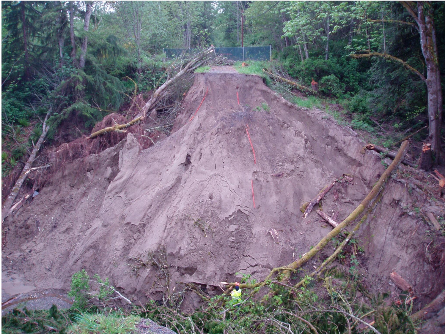
Figure 4b. Image of the damage to the Snoqualmie Valley Trail. Photo is looking across where the trail should connect across the stream in the bottom of the image. A King County employee is in the bottom center of the image wearing high-visibility green jacket. (Source: John Bethel. Accessed: 2017).
