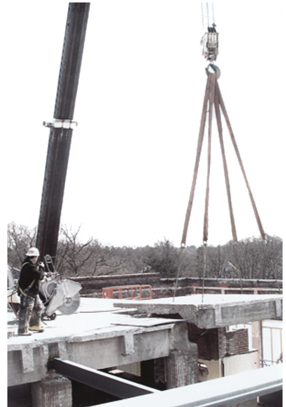
Figure 5.2.6_ Saw cutting and removal of structure
