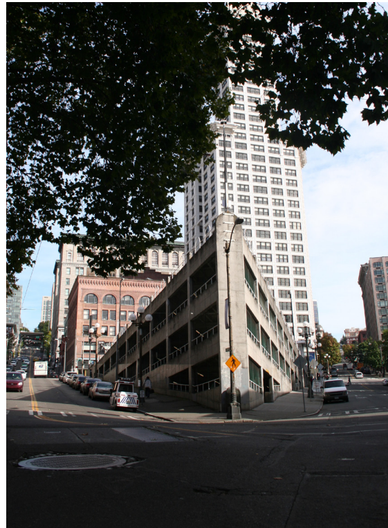
Figure 5.1.2_ 'Sunken Ship Parking Garage Existing structure viewed from pioneer square
