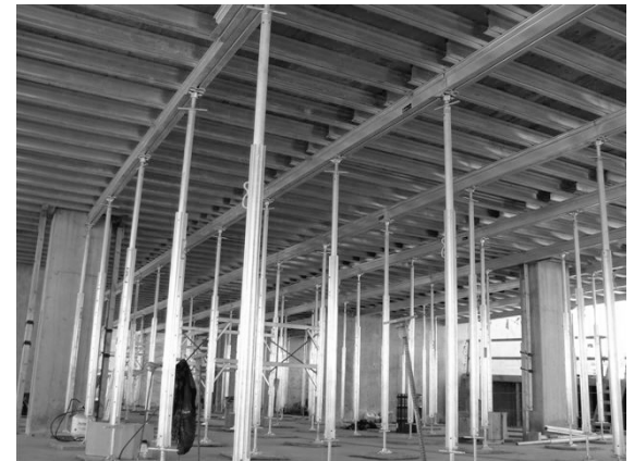
Figure 5.2.7_ Shoring of existing structure to remain
