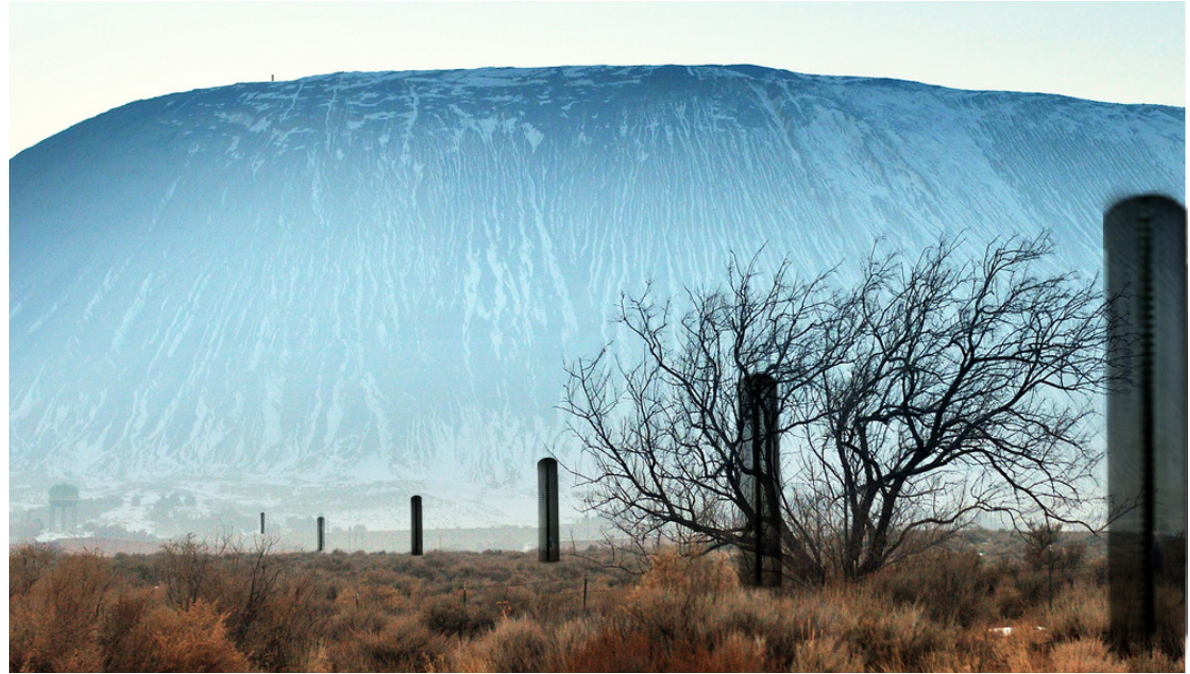
Figure 4.4.1 - Light-wells marking the tunnel on the landscape. Original photo courtesy of Ryan Houston
